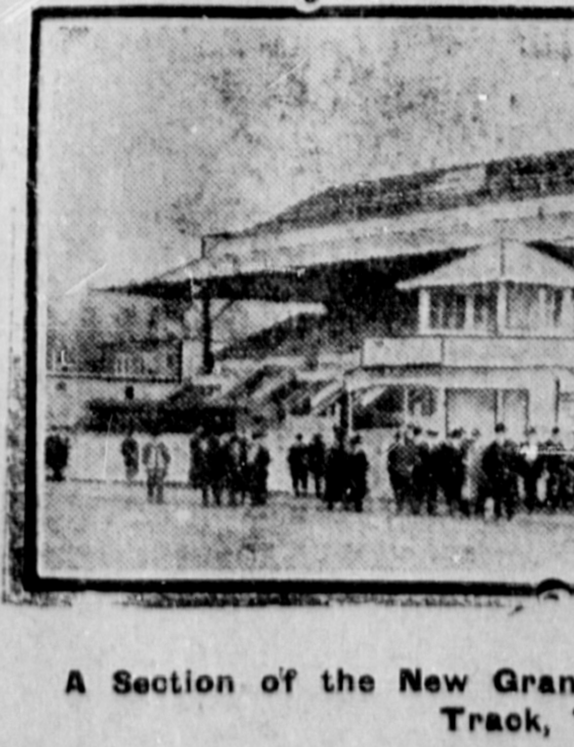
A Section of the new Grand Stand at the Woodbine Race Track, Toronto.
