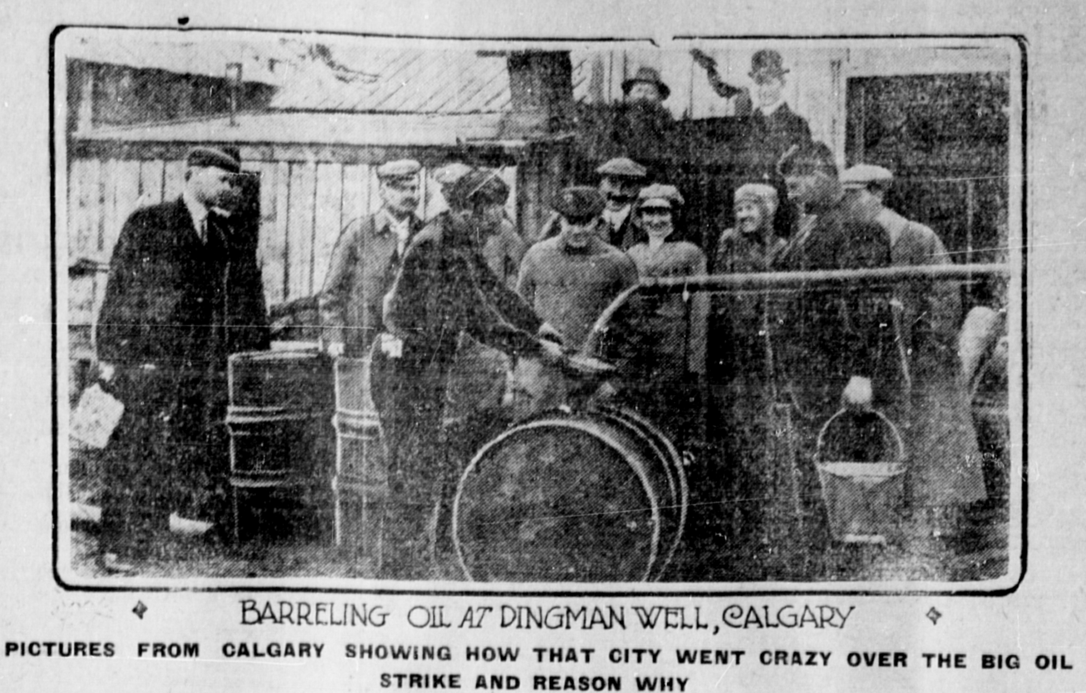
BARRELING OIL AT DINGMAN WELL, CALGARY. PICTURES FROM CALGARY SHOWING HOW THAT CITY WENT CRAZY OVER THE BIG OIL STRIKE AND REASON WHY
