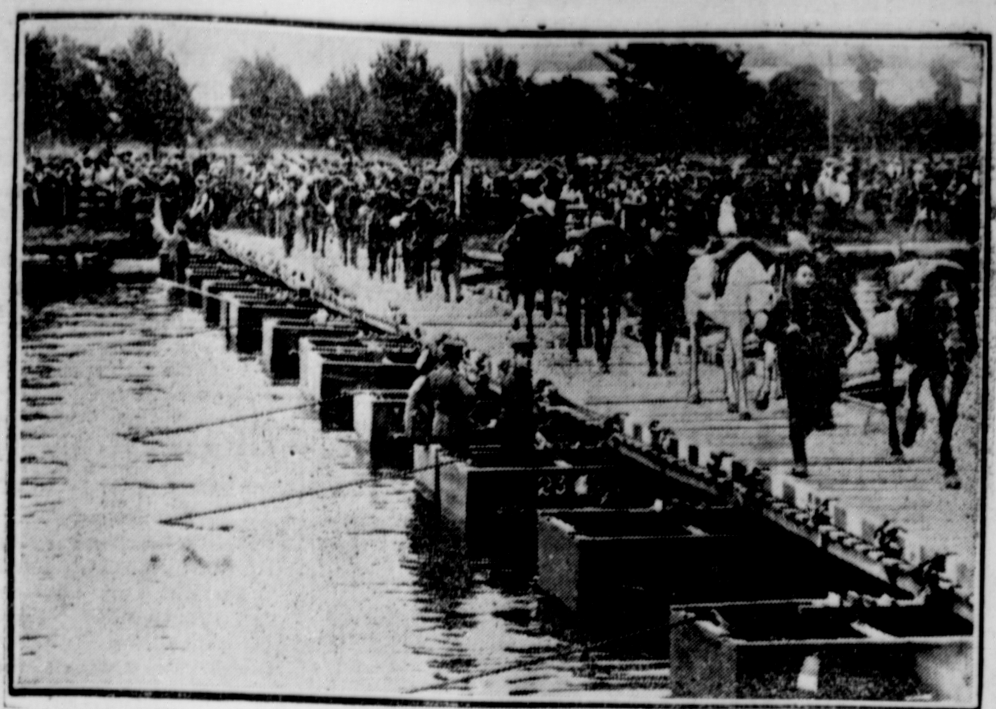
PONTON BRIDGE CONSTRUCTED BY THE ROYAL BRITISH ENGINEERS. This is a bridge such as the British army will use to cross a good many streams in Belgium. Cavalry is shown going over the one that appears in the picture.
