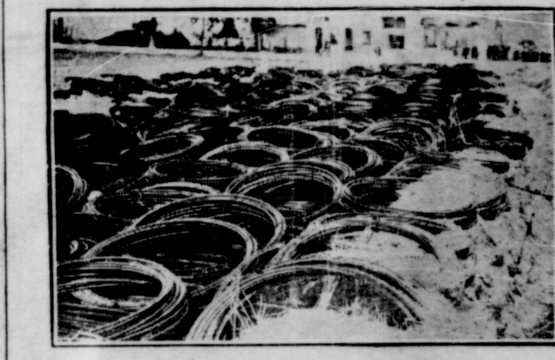
PROTECTION FOR GERMAN TRENCHES The Germans have found a new plan for the protection of their soldiers in the trenches. Coils of wire are placed before the trenches and when a shell falls they prevent the fragments from spreading to the trenches.
