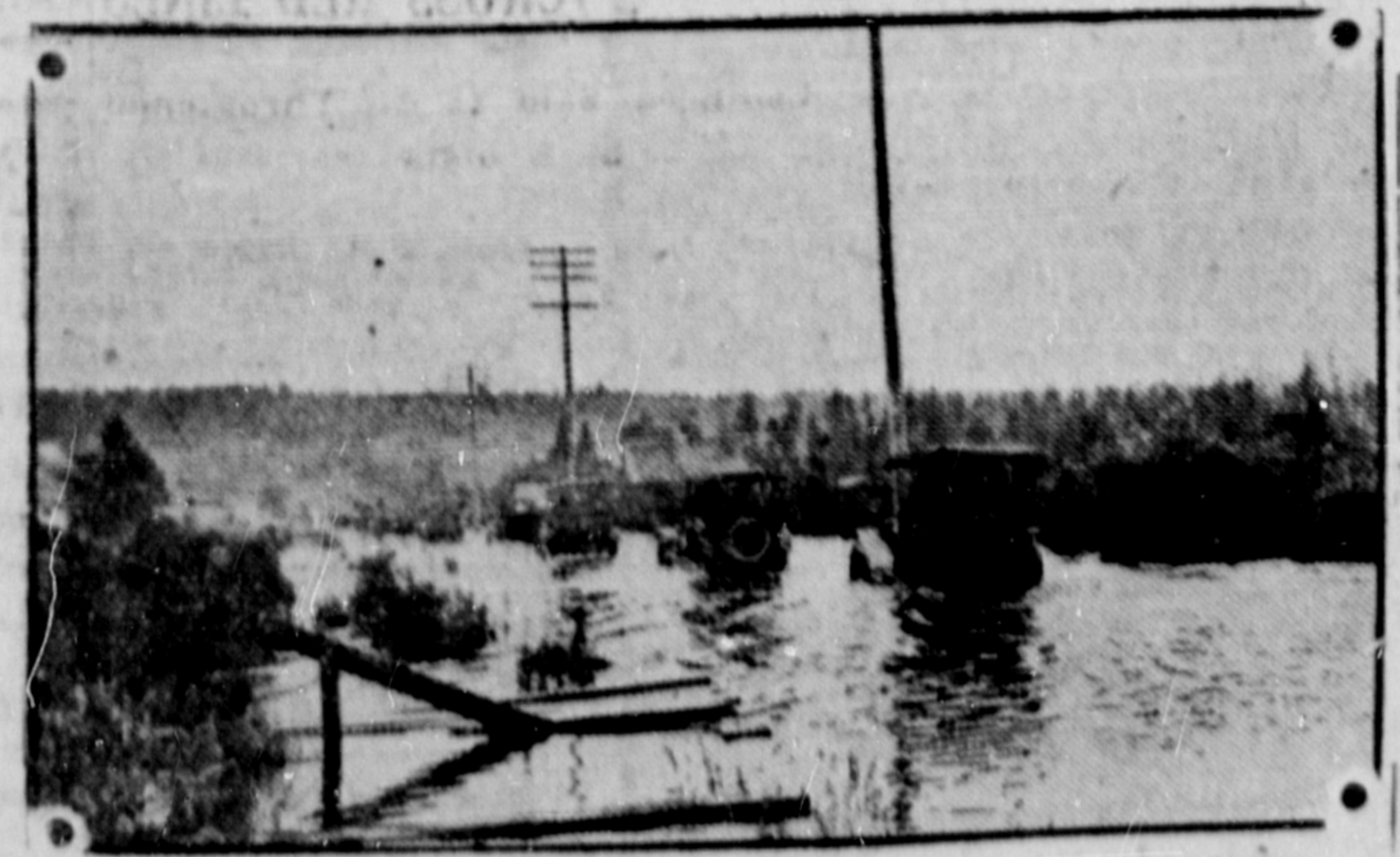
Automobiles up to axles in water at the approach to the bridge over the Fraser River at New Westminster during the recent freshets.
