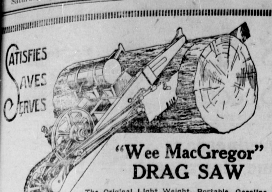
The Original Light Weight, Portable, Gasoline Operated Drag Saw and Power Plant.
