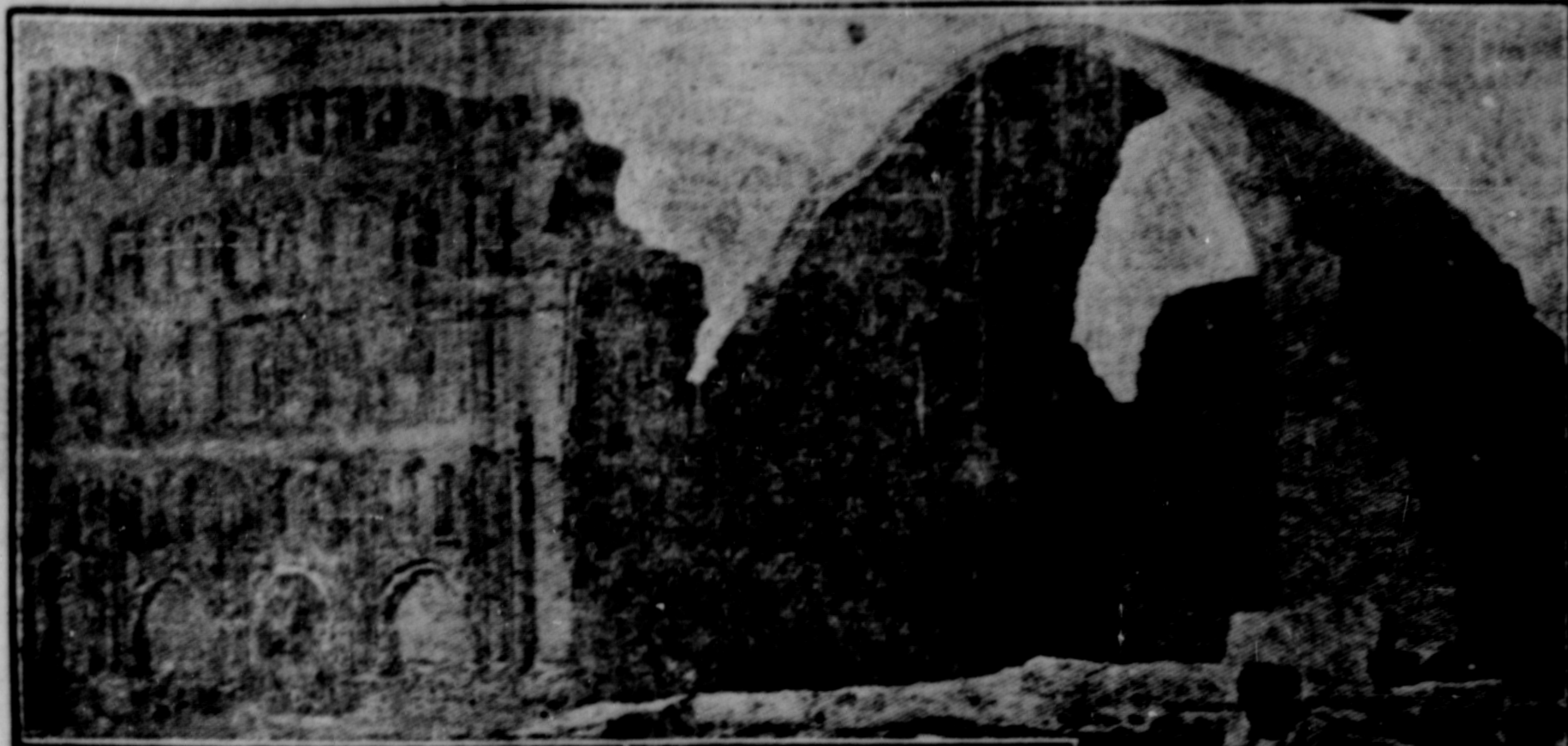
PICTURESQUE RUINS OF CTESIPHON.—These date back to the sixth century. This is a photograph of the ruined palace. The huge arch of the hall shown above is 83 feet wide by 95 feet high, and the walls are 23 feet wide at their base. The arch is built of brick baked more than thirteen hundred years ago.
