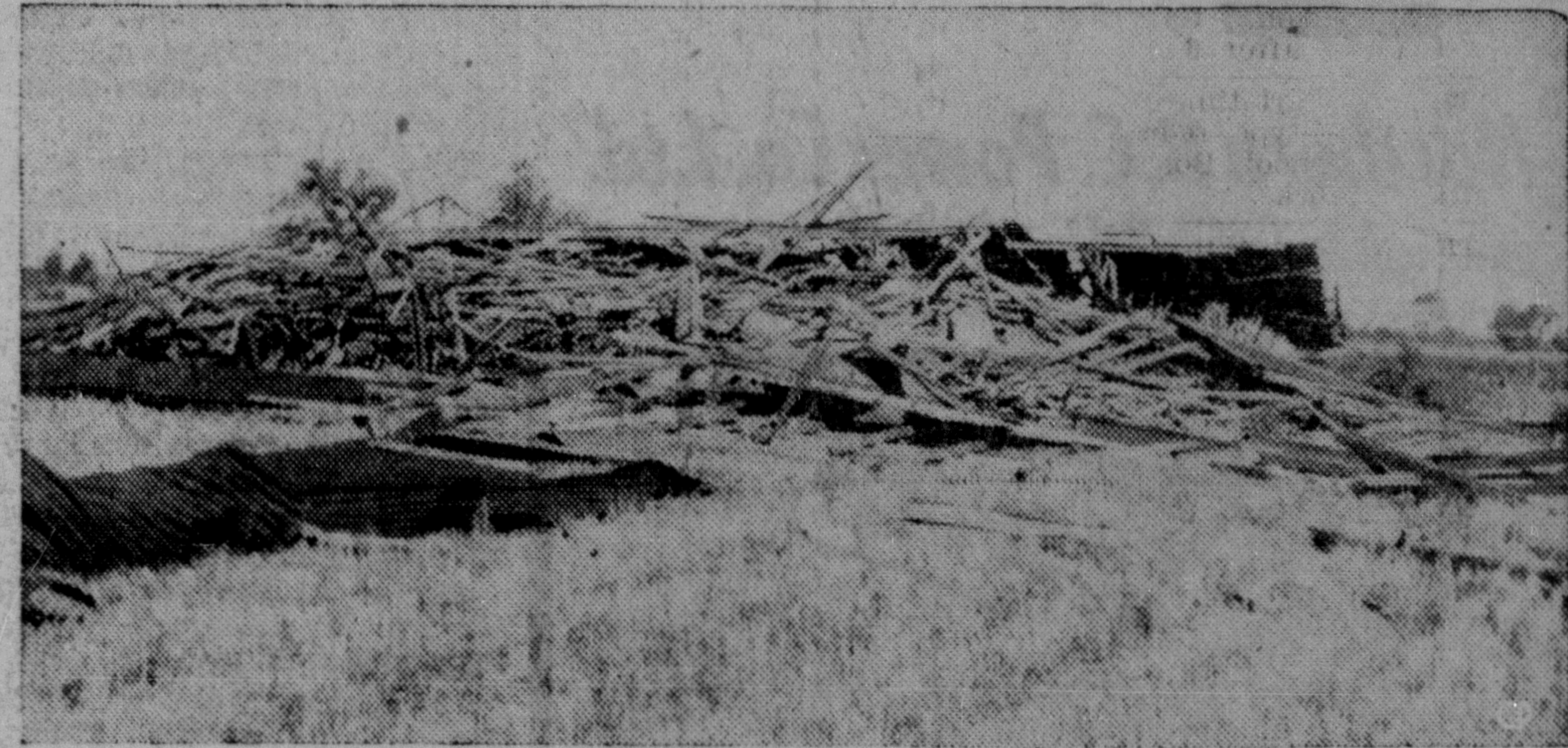
TORNADO STRIKES —Three barns were wrecked and several damaged by a tornado which struck near Chatham, Ont., causing damage estimated at several thousand dollars. Trees were uprooted, highways blocked, and power and telephone lines levelled in the path of the twister, a mile wide and five miles long. This pile of splintered wood was formerly the barn of Morton Wickwire. (CP PHOTO)
