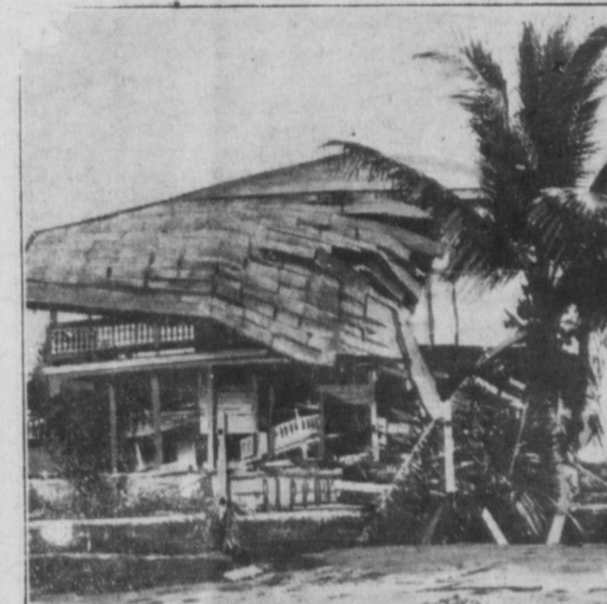
One of the scores of dwellings in Cuyutlan, Mexico, where many were recently killed and injured when 'quake and tidal wave wrecked every building in the town. Most of victims were children at play on the beach.
