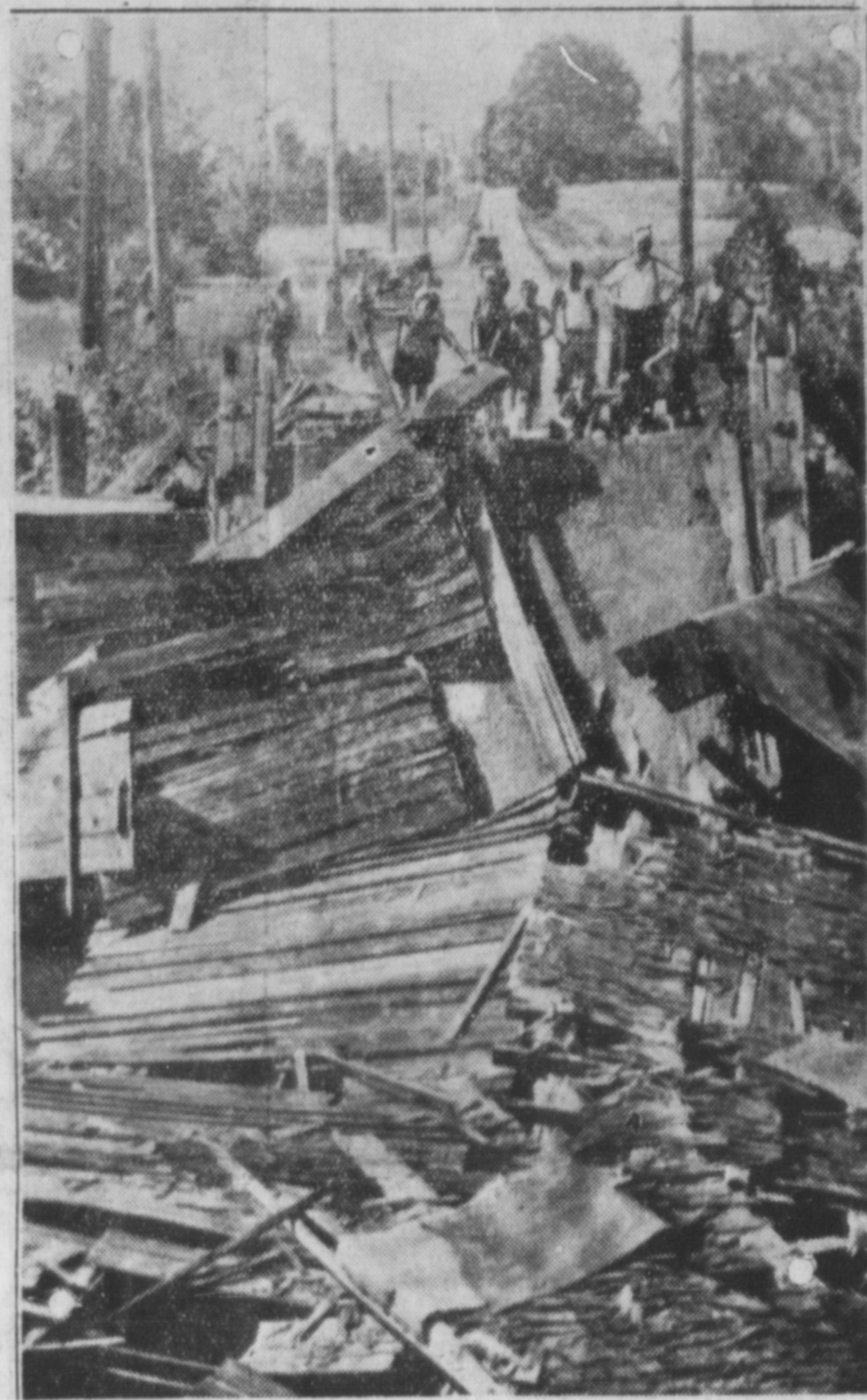
Imagine his embarrassment. A truck driver was half way across this ancient covered bridge at Greenfield, Mass., when it started to sag. He stepped on the gas. Just made it
