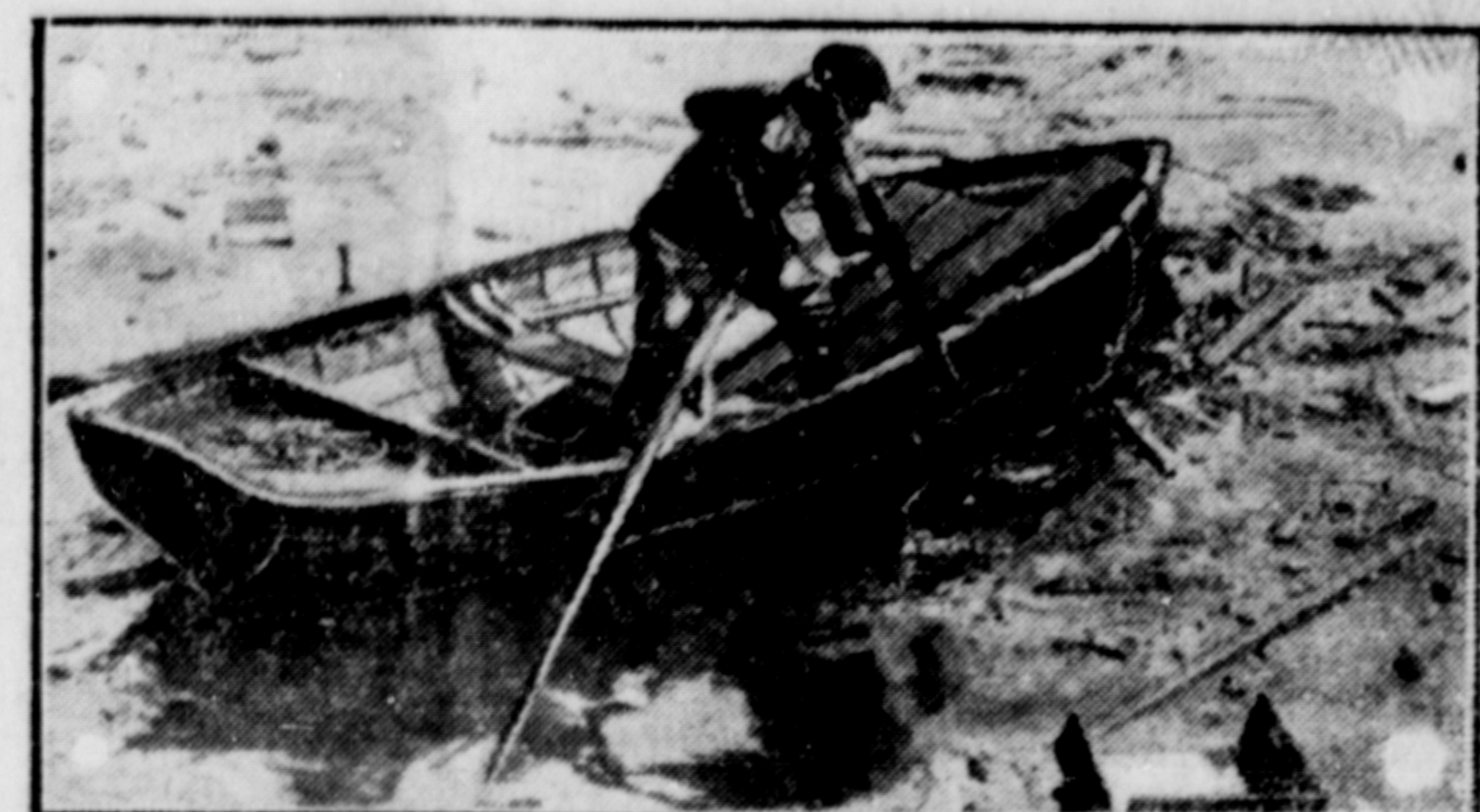
Boatmen in Southampton reap a good harvest from the old fittings and woodwork left floating near the dock after the departure of big liners.
