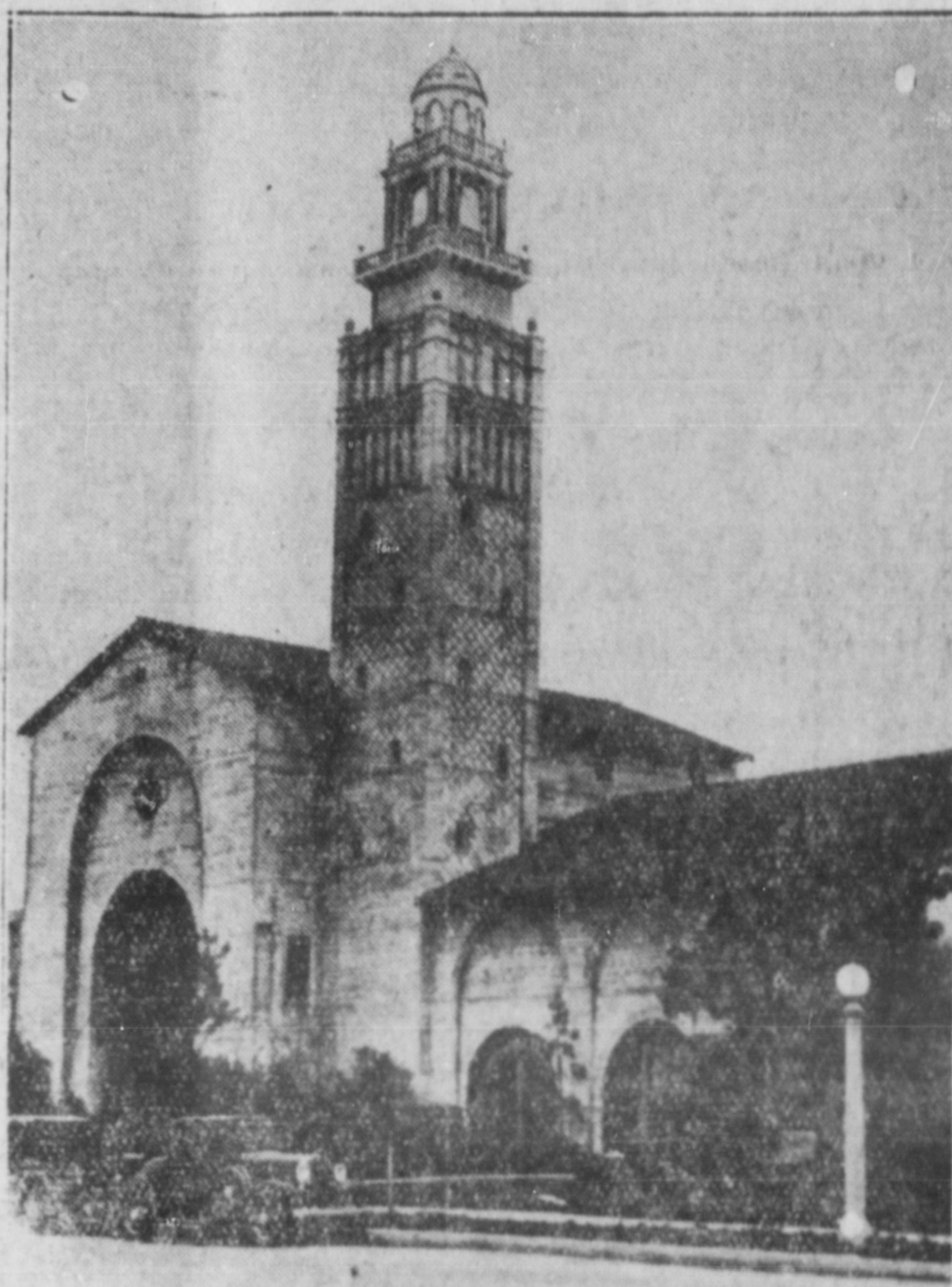
Three guesses and you're still wrong. No church, home or city hall this but the swanky sewage disposal plant of Beverly Hills, California, where the grand manner is applied to all things.
