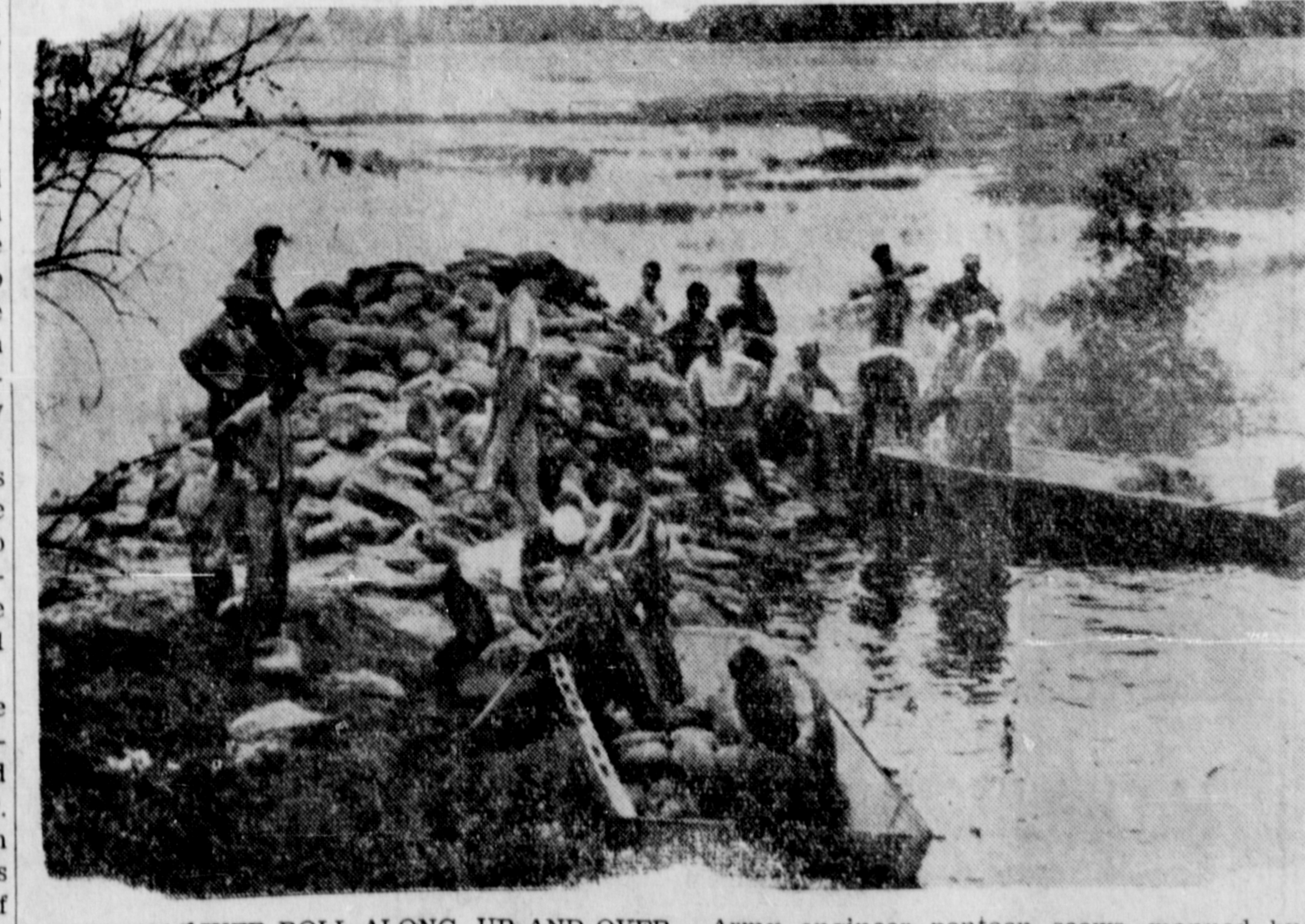
OL' MAN RIVER ROLL ALONG, UP AND OVER—Army engineer pontoon scows, manned by civilian volunteers, are pictured bringing sandbags to levees on the Mississippi River to bolster the already-weakened levees. Convergence of the Mississippi and Missouri Rivers have caused the highest floods since 1844.
