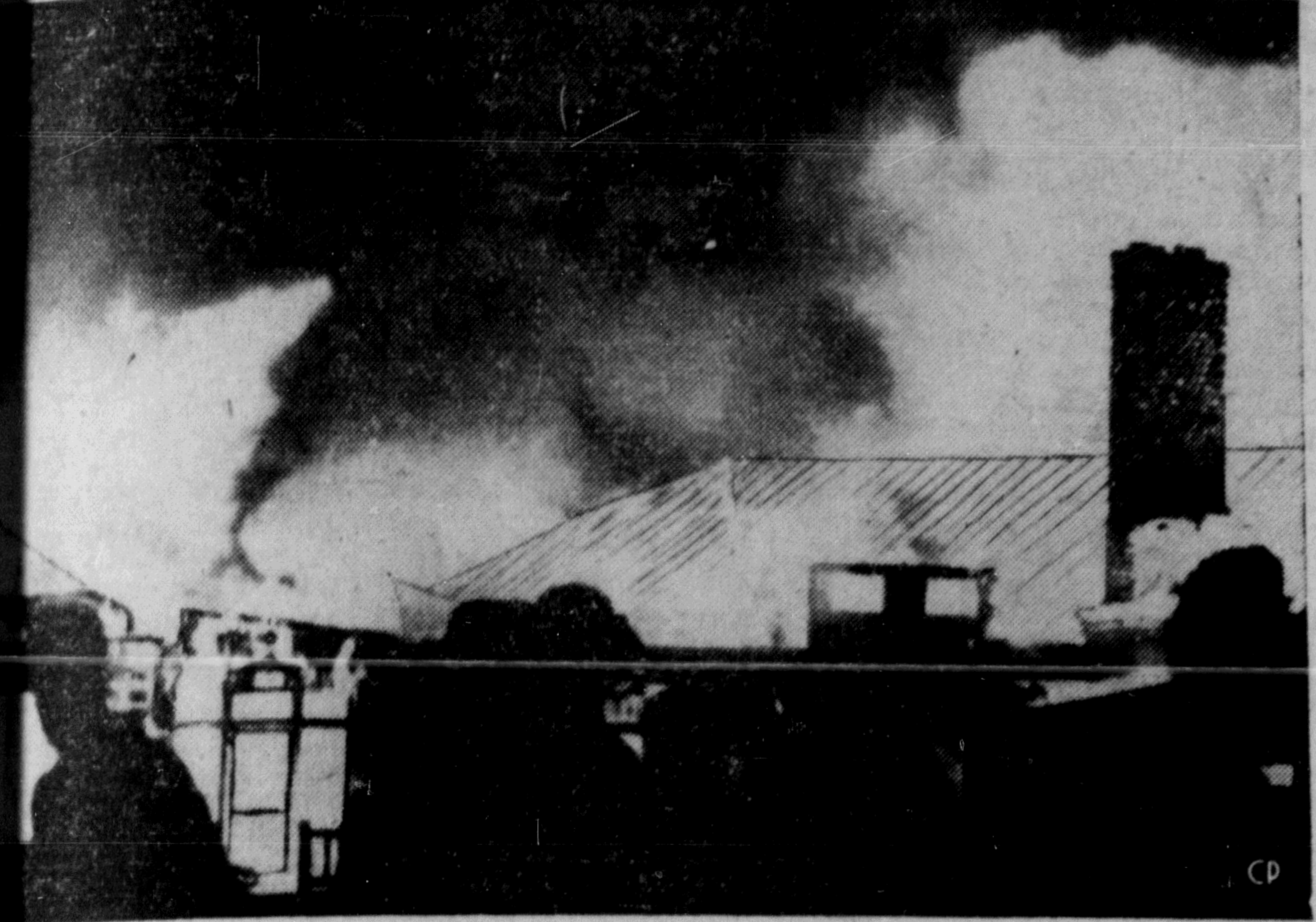
1,000 FIRE —Flames race through the main ballroom of luxurious Jasper Park Lodge, 225 miles west of Edmonton. Shortly before, 300 persons had been dancing in what was reputed to be the largest log building in the world. Damage is estimated at about $1,000,000 by the Canadian National Railways, which owns the summer resort. The three-storey lodge, built in 1922, was destroyed. The fire is believed to have started near the check-room in the administration wing. (CP PHOTO)
