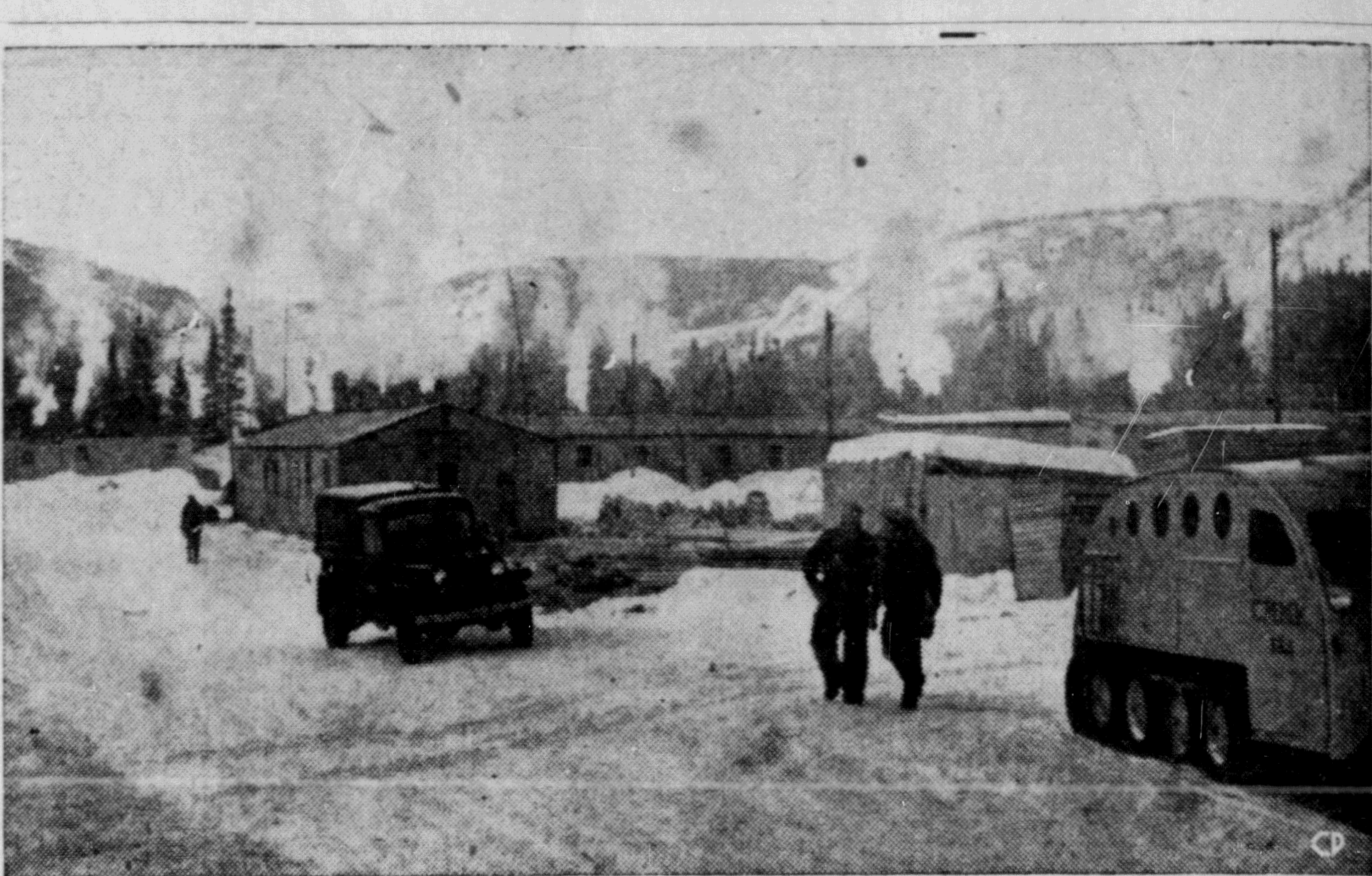
WINTER CAMP—Temperatures fall as low as 30 below zero in Labrador-Ungava but construction of the 360-mile railway to Seven Islands, Que., goes on. Some members of a day shift leave the warm shelter of their huts in the winter railway camp for work. (CP PHOTO)
