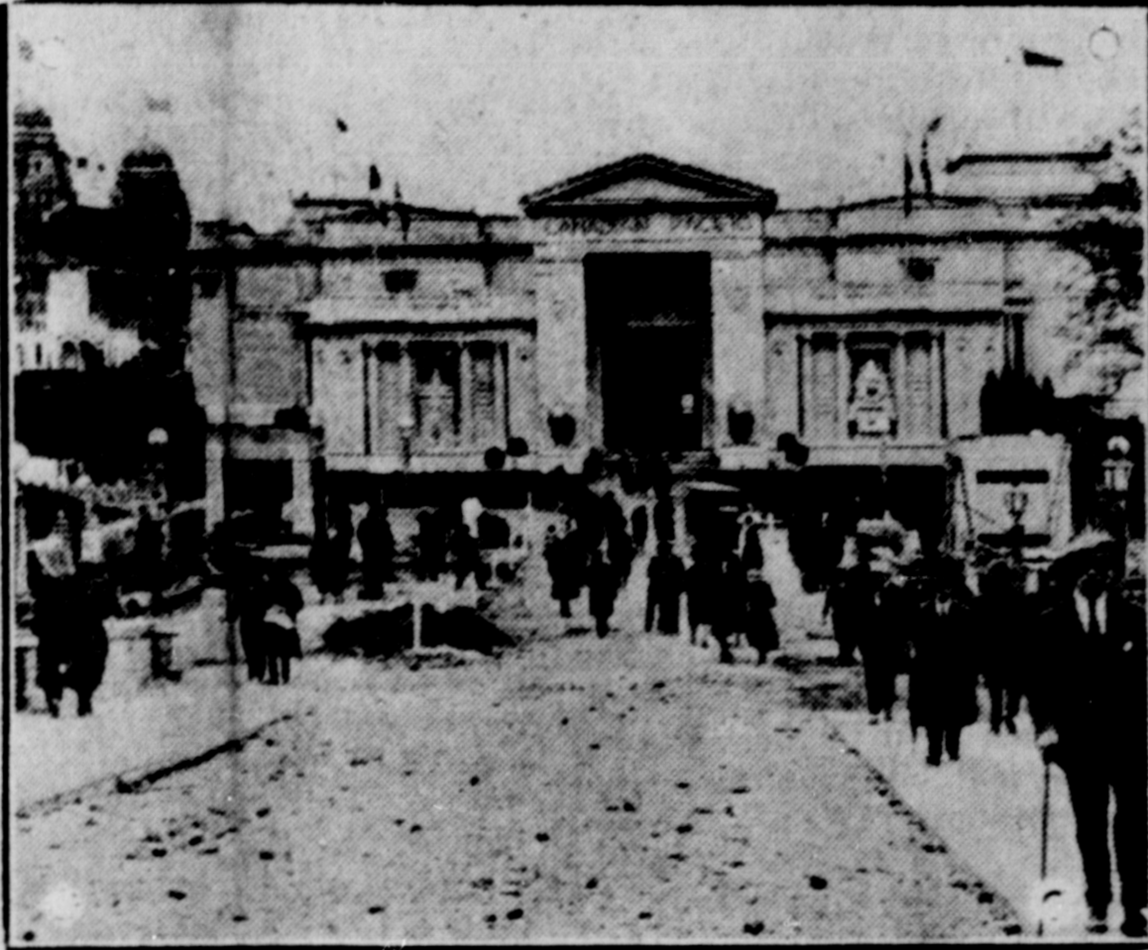
Looking from Old London Bridge, this is the way the Canadian Pacific building shows up at the British Empire Exposition. A few construction debris remain to be cleared away, but otherwise the building is complete, as pictured
