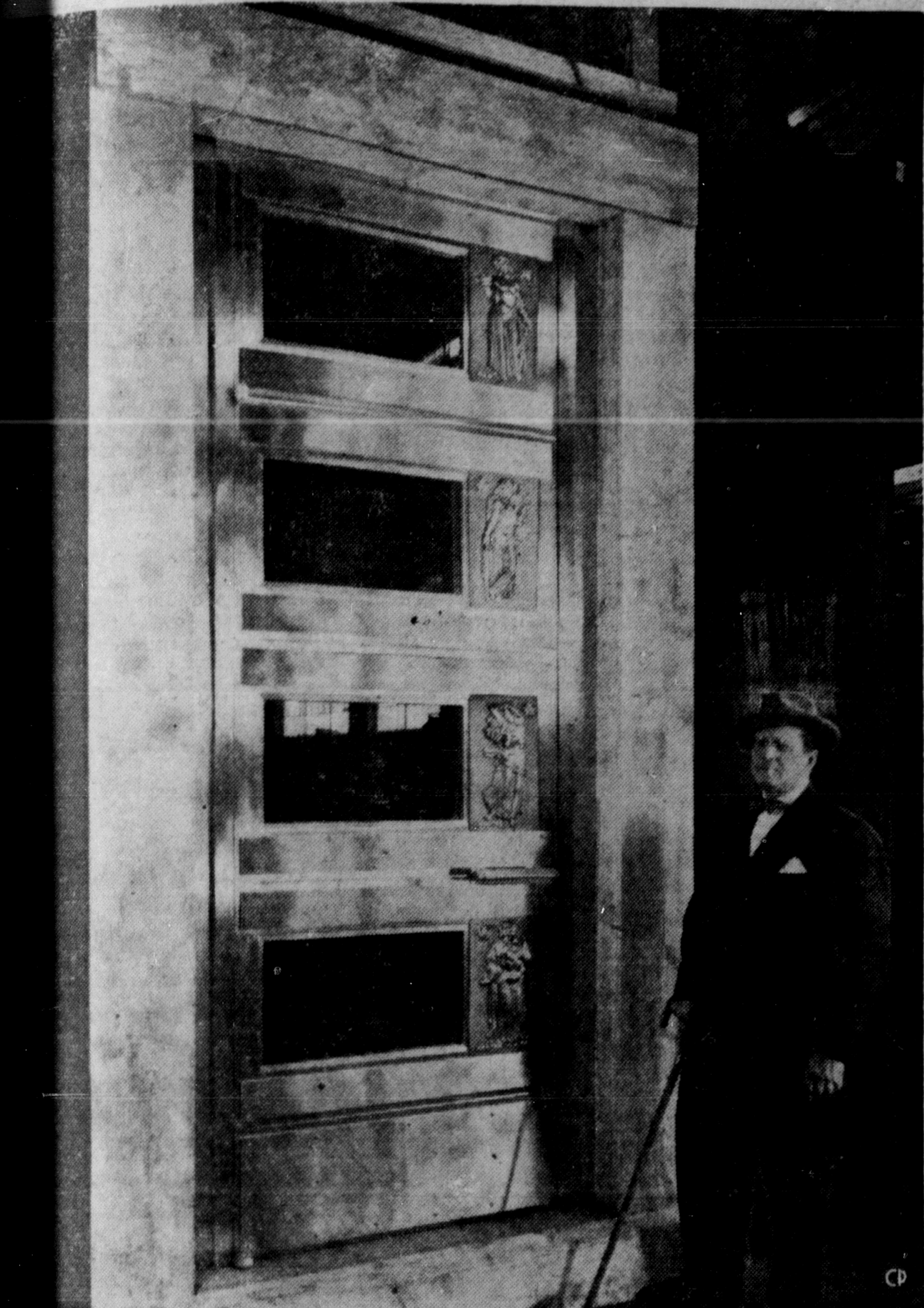
GIFT—Canada's contribution to the United Nations' general assembly building headquarters in New York are seven doors, designed by a Canadian and using Canadian metal. A special alloy of copper, zinc and nickel was created for the doors, each of which is six inches high, 40 inches wide and valued at $10,000. Architect Ernest Corbett, Montreal, designer, is at right. (CP PHOTO)
