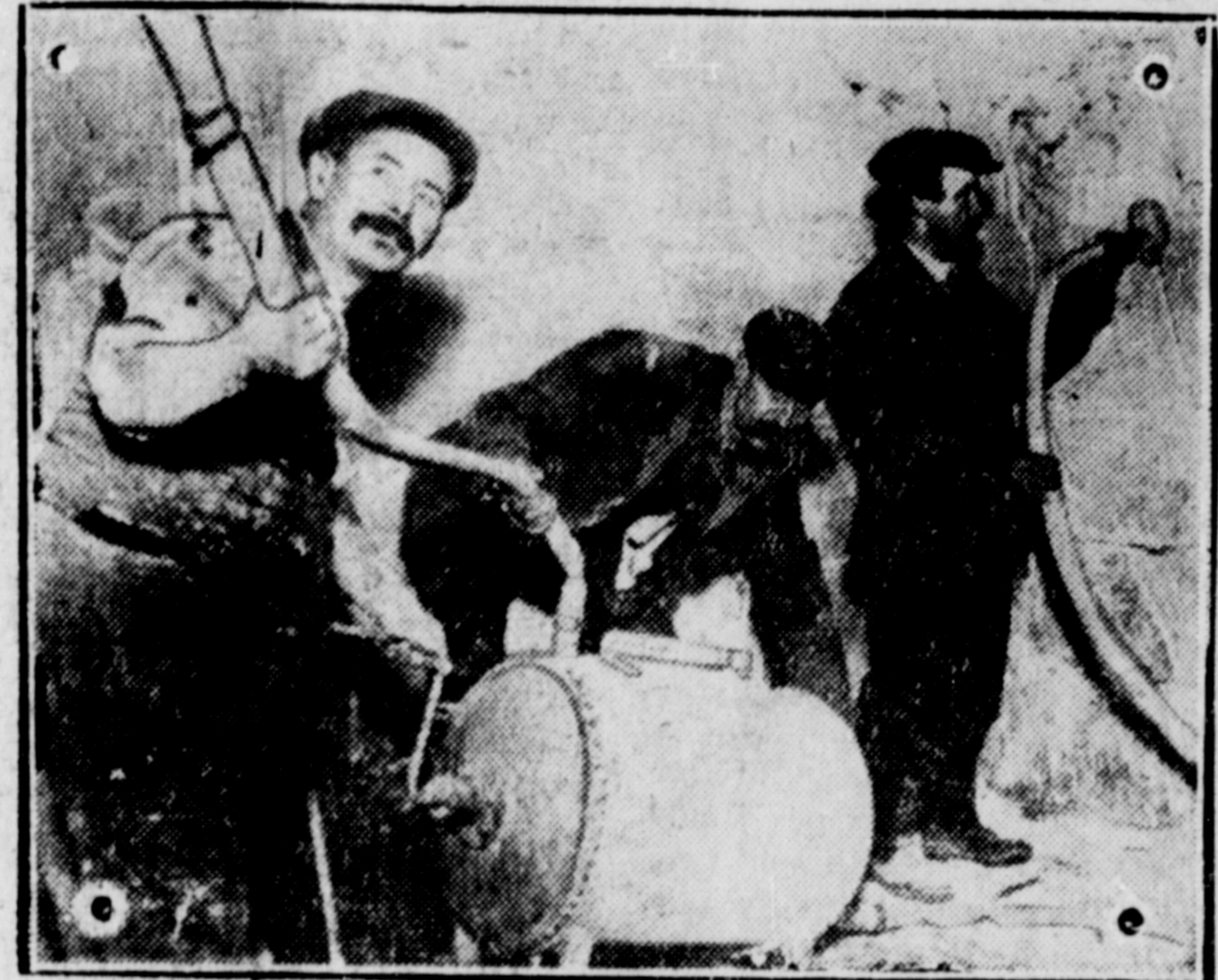
Workmen are filling the cracks in the dome of the new St. Paul's Cathedral, London, with compressed cement in their effort to save the towering edifice that has overlooked the city for so many years.
