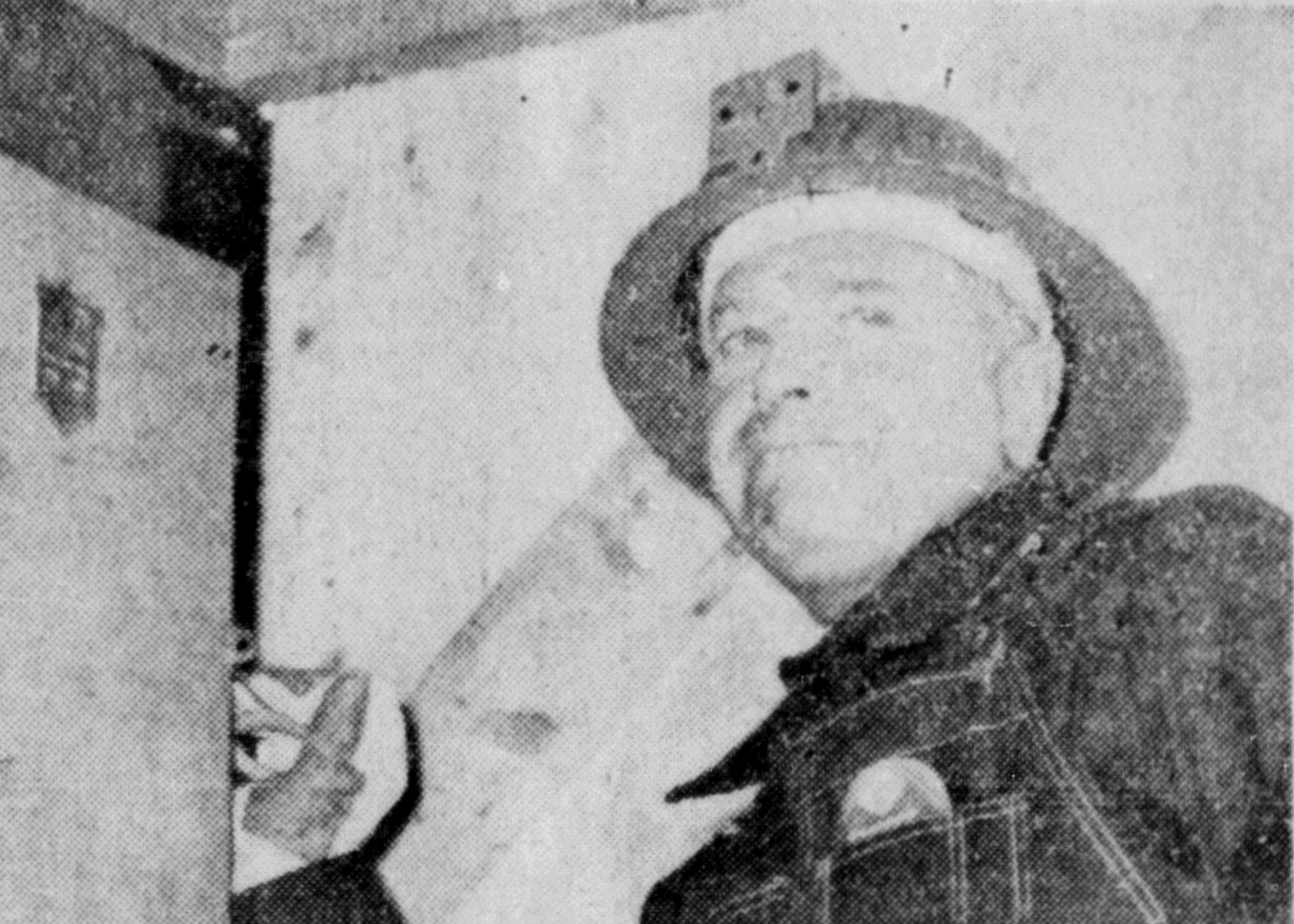
SETS OFF BLAST —One of Canada's biggest construction jobs, the $22,750,000 Strait of Canso causeway from Cape Breton to the mainland, was officially set in motion at Auld's Cove, N.S., when Transport Minister Chevrier pulled a switch. He set off eight tons of dynamite which tore away 40,000 tons of rock and earth from centuries-old Porcupine Mountain, the source of supply for the causeway fill. (CP PHOTO)
