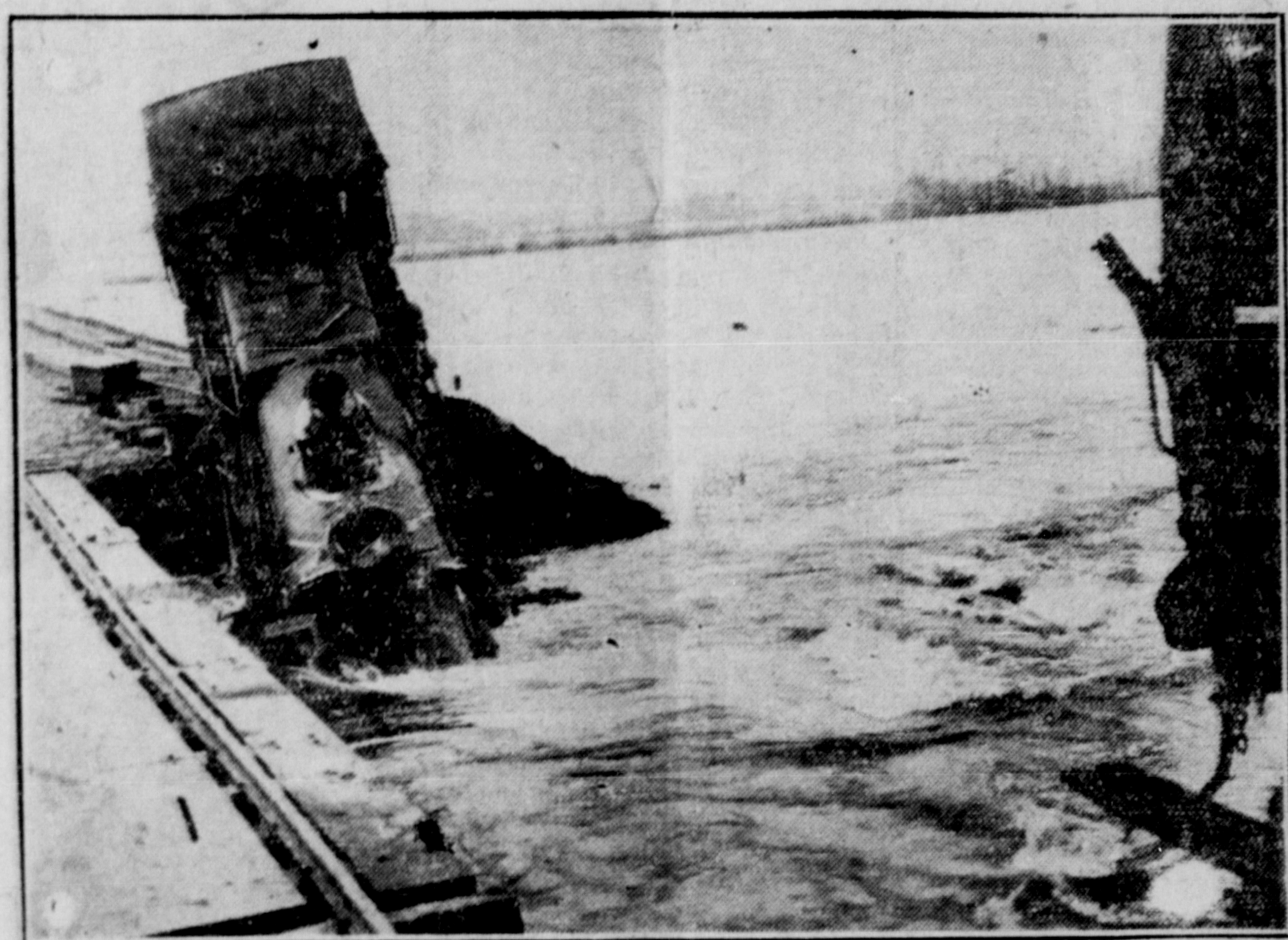
DYKE BREAK CAUSES TRAIN WRECK—The above graphic photo illustrates one of the terrible results of the breaking of a dyke near Beugen, Holland. The tracks were washed away and the speeding train was derailed into the water. Floods in Holland are said to have caused more damage than any other similar disaster in years.
