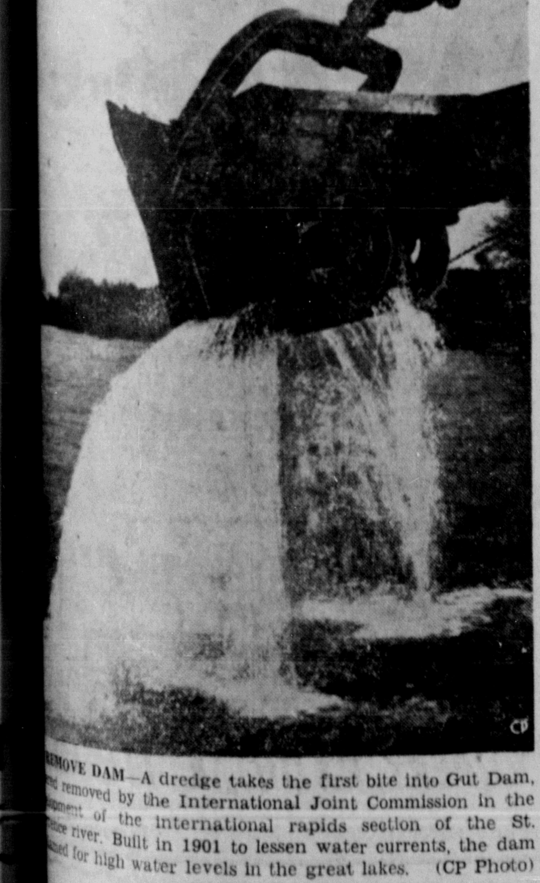
REMOVE DAM —A dredge takes the first bite into Gut Dam, removed by the International Joint Commission in the interest of the international rapids section of the St. Lawrence river. Built in 1901 to lessen water currents, the dam caused high water levels in the great lakes. (CP Photo)
