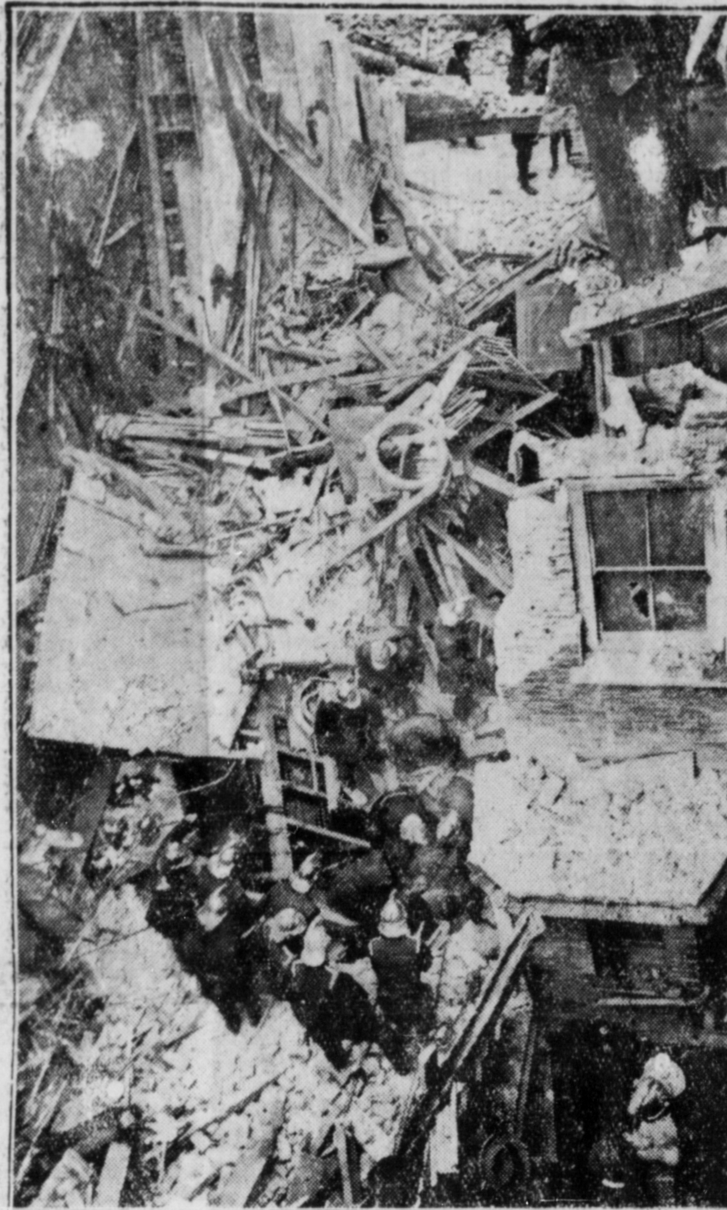
REGENT STREET BUILDING COLLAPSES: Firemen searching debris of house and shop in Beak Street, off Regent Street, in the heart of London's West End.
