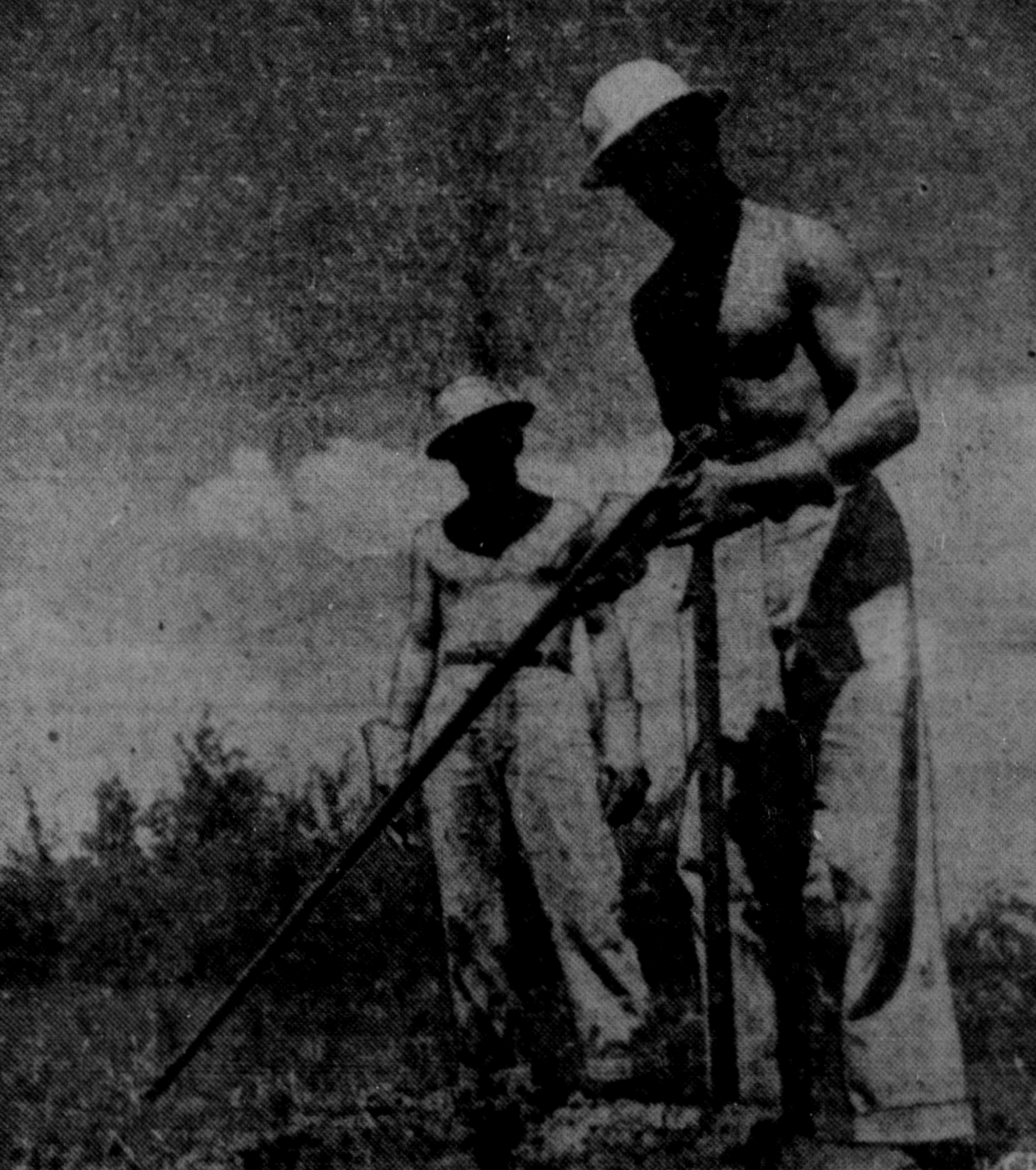
MAKE EARTHQUAKE —Modern methods of searching for oil use highly-developed technical skills. These workmen are members of a seismic party. They are tamping down a charge of dynamite placed in a hole, to create a miniature, artificial earthquake. The vibrations caused in the earth are recorded on sensitized paper by instruments on a nearby truck. A study of these reveals whether the area is promising. (CP Photo)
