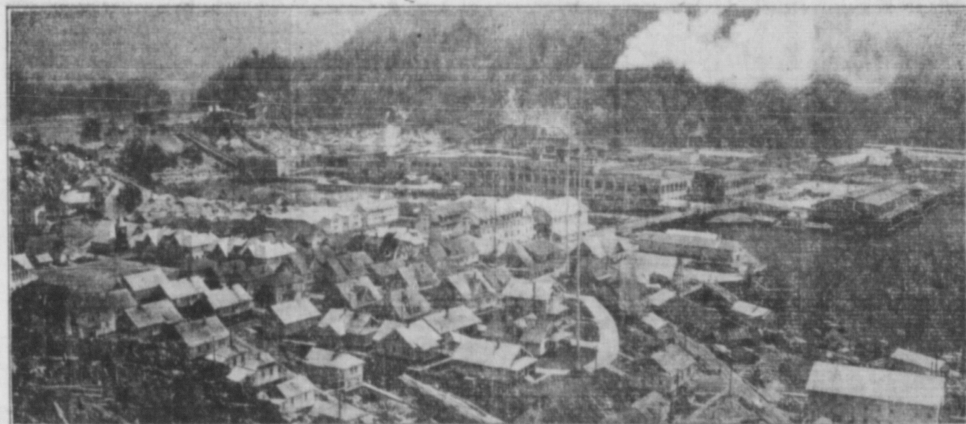
OCEAN FALLS—Paper mill, one of largest producers in this district.
