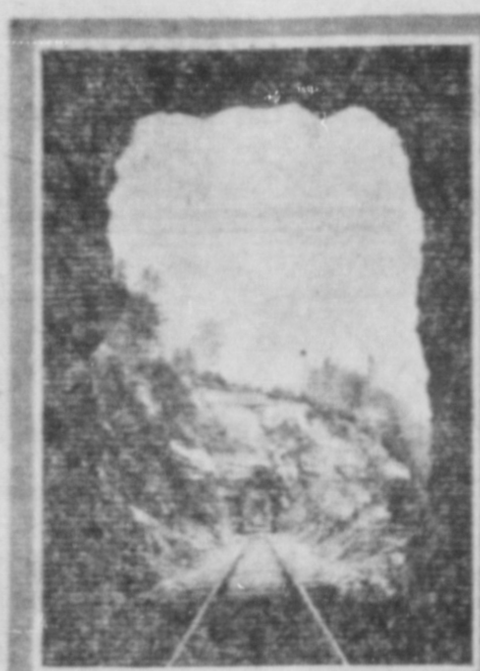
The Three Tunnels at Kiplin Canyon on G.T.P.
