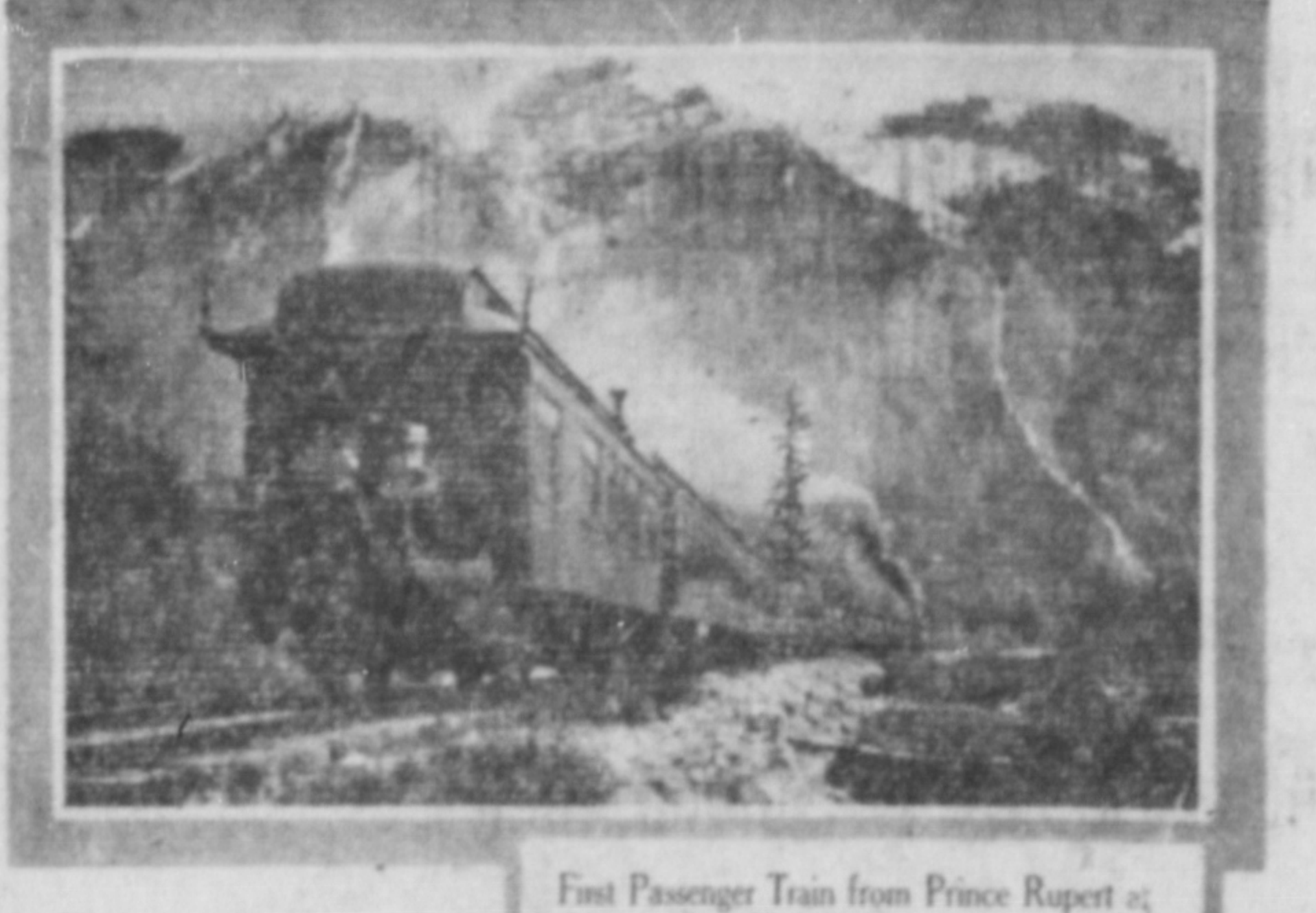
First Passenger Train from Prince Rupert at Mile 45—June 14, 1911
