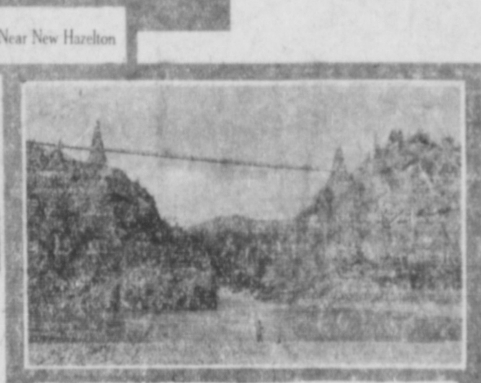
Bridge across Bulkley River Near New Hazelton 600 ft. long; 260 ft. high; 9 ft. wide
