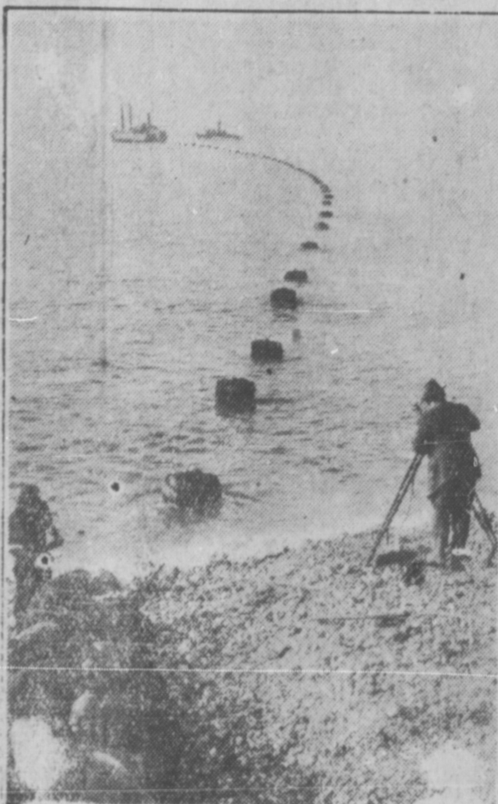
LAYING THE LAST LINK of direct cable from France to America. The S.S. Colonia connecting La Havre, France and Penzance, England, where the present cable ends
