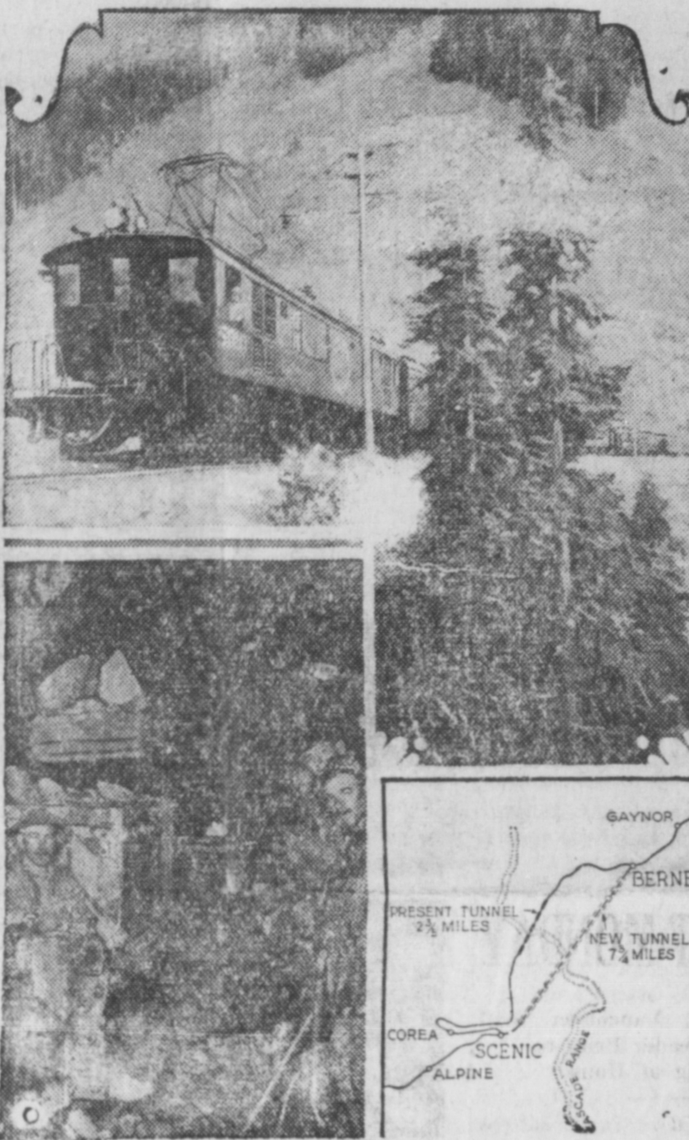
Above is a layout showing (top) one of the new electric trains about to enter the Cascades tunnel; drillers at work inside the tunnel (bottom, left), while bottom, right, is a map which illustrates the old and the new routes through the range. This new tunnel, which is 7.79 miles long, was formally opened on January 12. It has cost more than $14,000,000 to construct, and it is the longest tunnel on the American continent.
