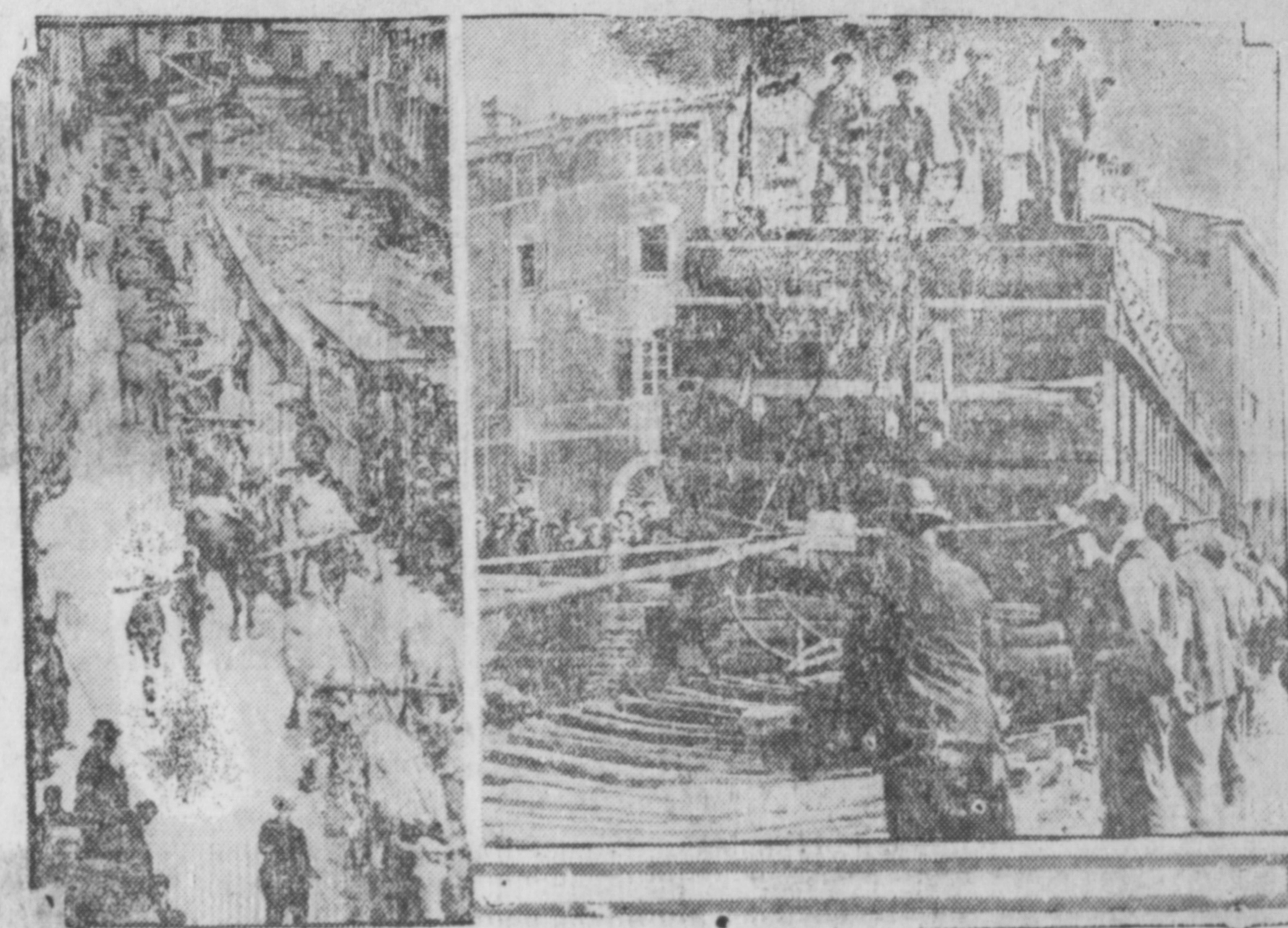
FIVE YEARS UNCEASING LABOR NEARLY DONE
