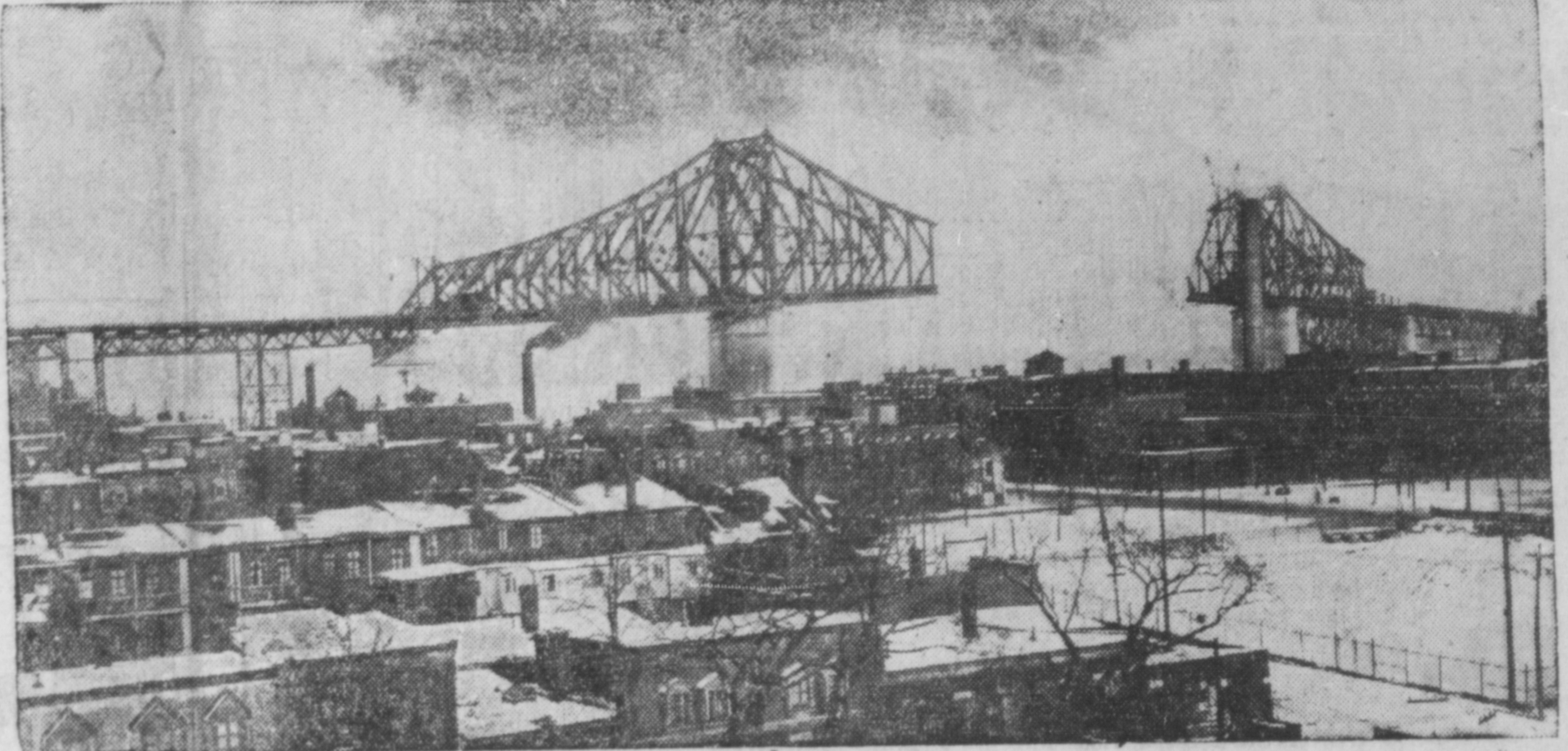
GREAT CANADIAN BRIDGE NEARS COMPLETION
