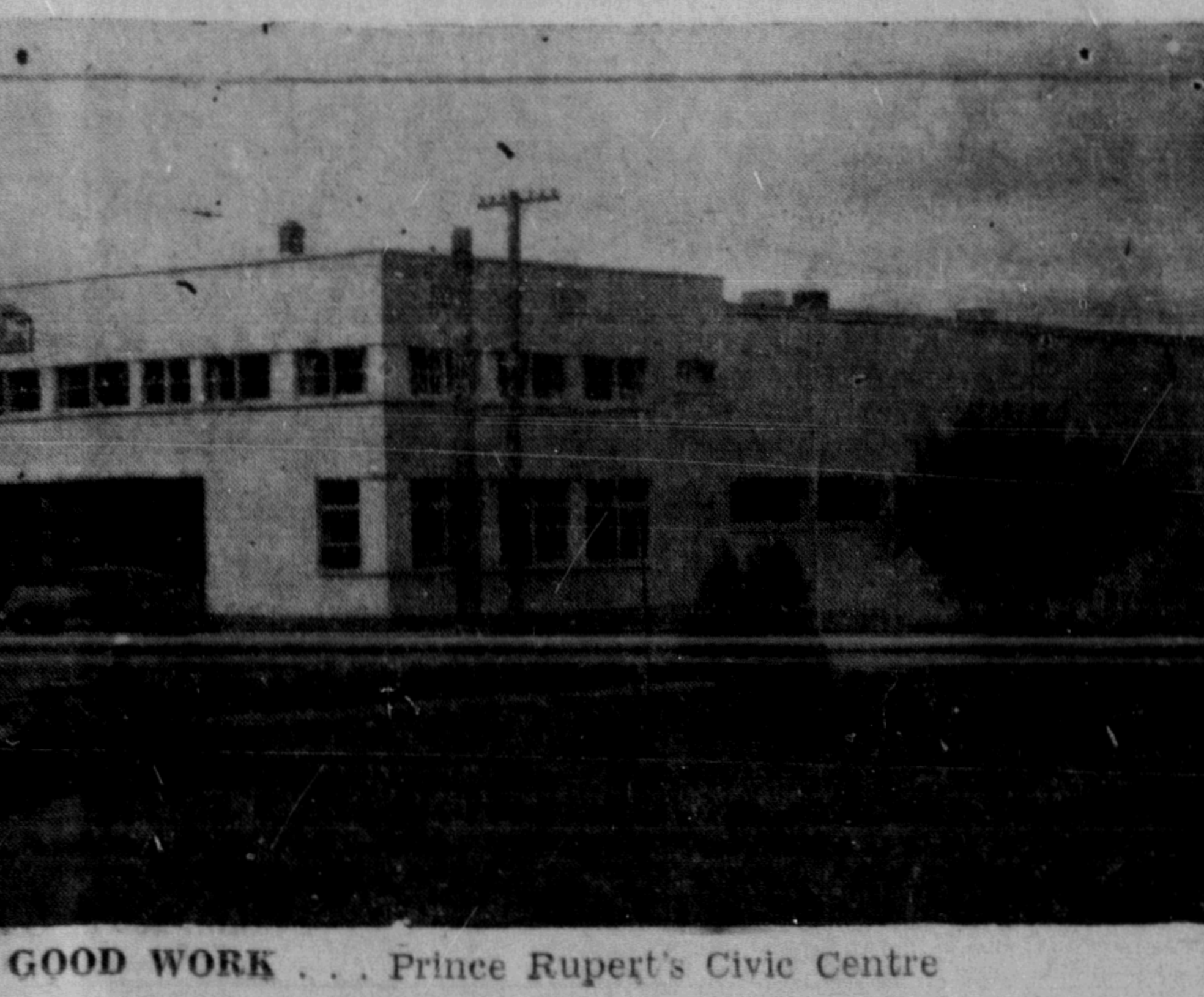
CONTINUES GOOD WORK . . . Prince Rupert's Civic Centre
