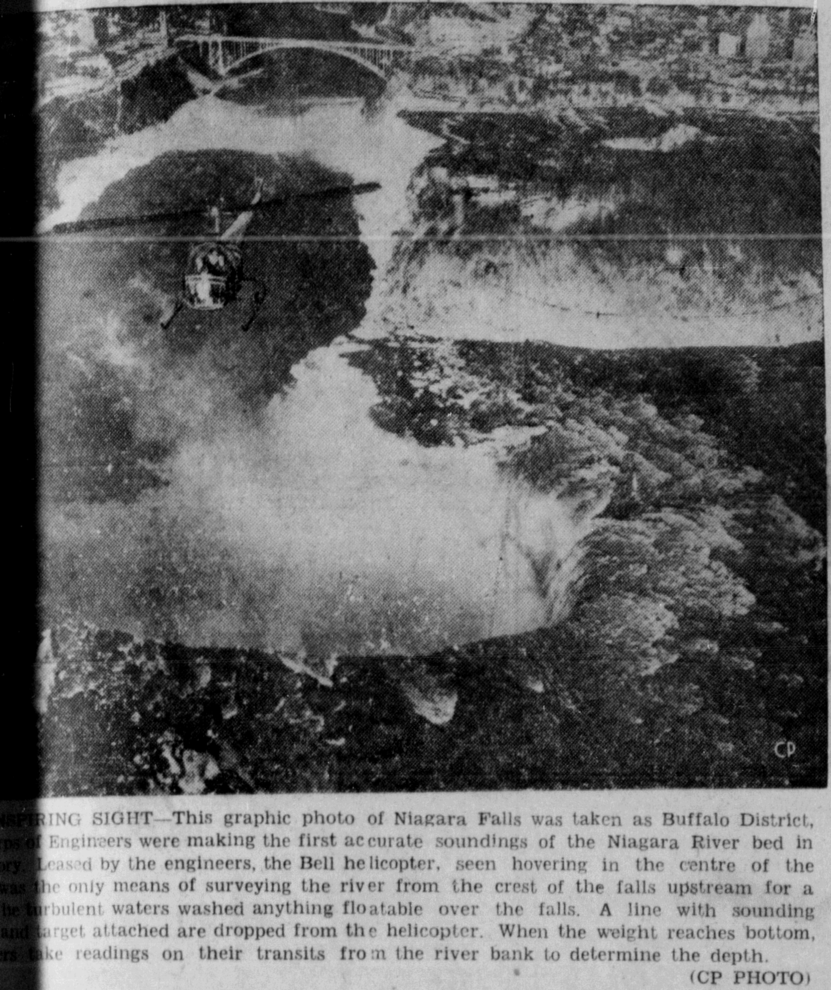
INSPIRING SIGHT—This graphic photo of Niagara Falls was taken as Buffalo District, Engineers were making the first accurate soundings of the Niagara River bed in the only means of surveying the river from the crest of the falls upstream for a turbulent waters washed anything floatable over the falls. A line with sounding and target attached are dropped from the helicopter. When the weight reaches bottom, take readings on their transits from the river bank to determine the depth. (CP PHOTO)
