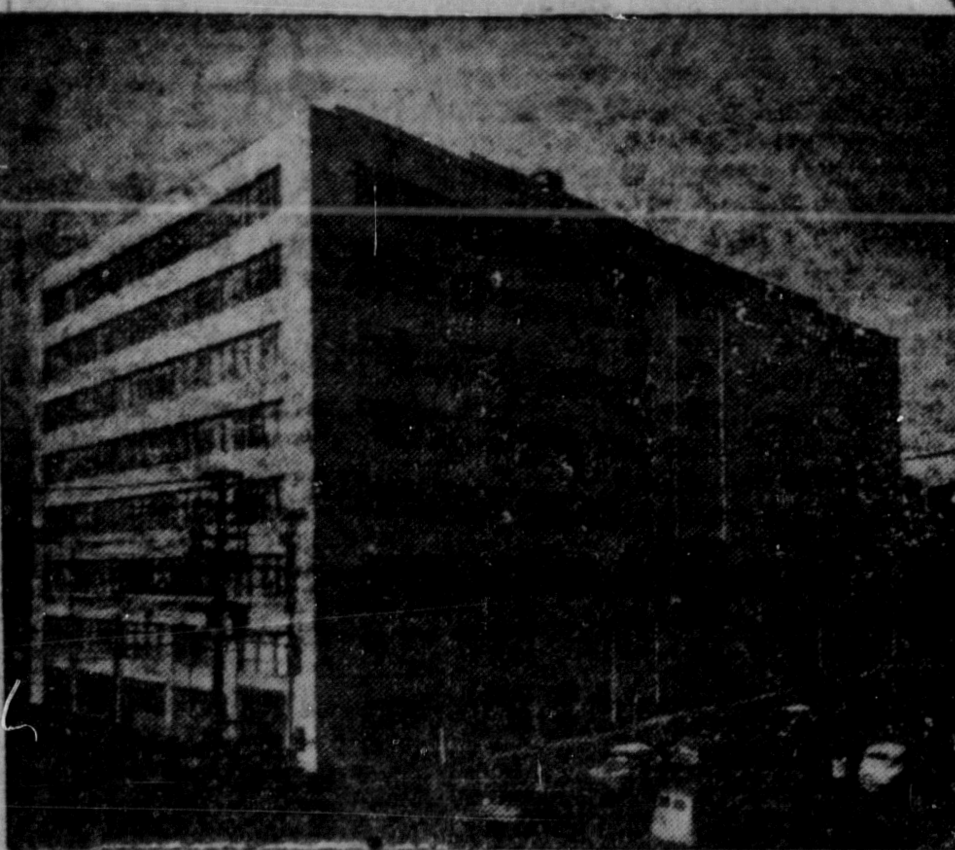
NEW TORONTO BUILDING—The British American Oil Co. has erected an eight-storey reinforced concrete building standing at the corner of Bay and College Streets, Toronto. It is the permanent home of more than 650 employees of Head Office and Central Region—the Ontario sales organization. Building dimensions are approximately 215 feet by 110 feet enclosing 2,500,000 cubic feet of space. The structure consists of a basement, ground floor, mezzanine, six full floors and penthouse. Flexibility and adaptability are the keywords and careful planning has ensured that every foot of space is utilized to the full. The building allows the whole of B-A's Toronto office staff to operate under one roof for the first time in a number of years. The closer co-ordination achieved will permit greater efficiency and more economical operation. The four top floors and the penthouse are occupied by B-A, other building tenants include James Lovick and Co., Advertising; The Continental Casualty Co.; The Bank of Toronto; Massie and Renwick, Insurance; Sun Life Assurance Company; The Agricultural Loans Division of the Ontario Government; and Murray's Restaurants.
