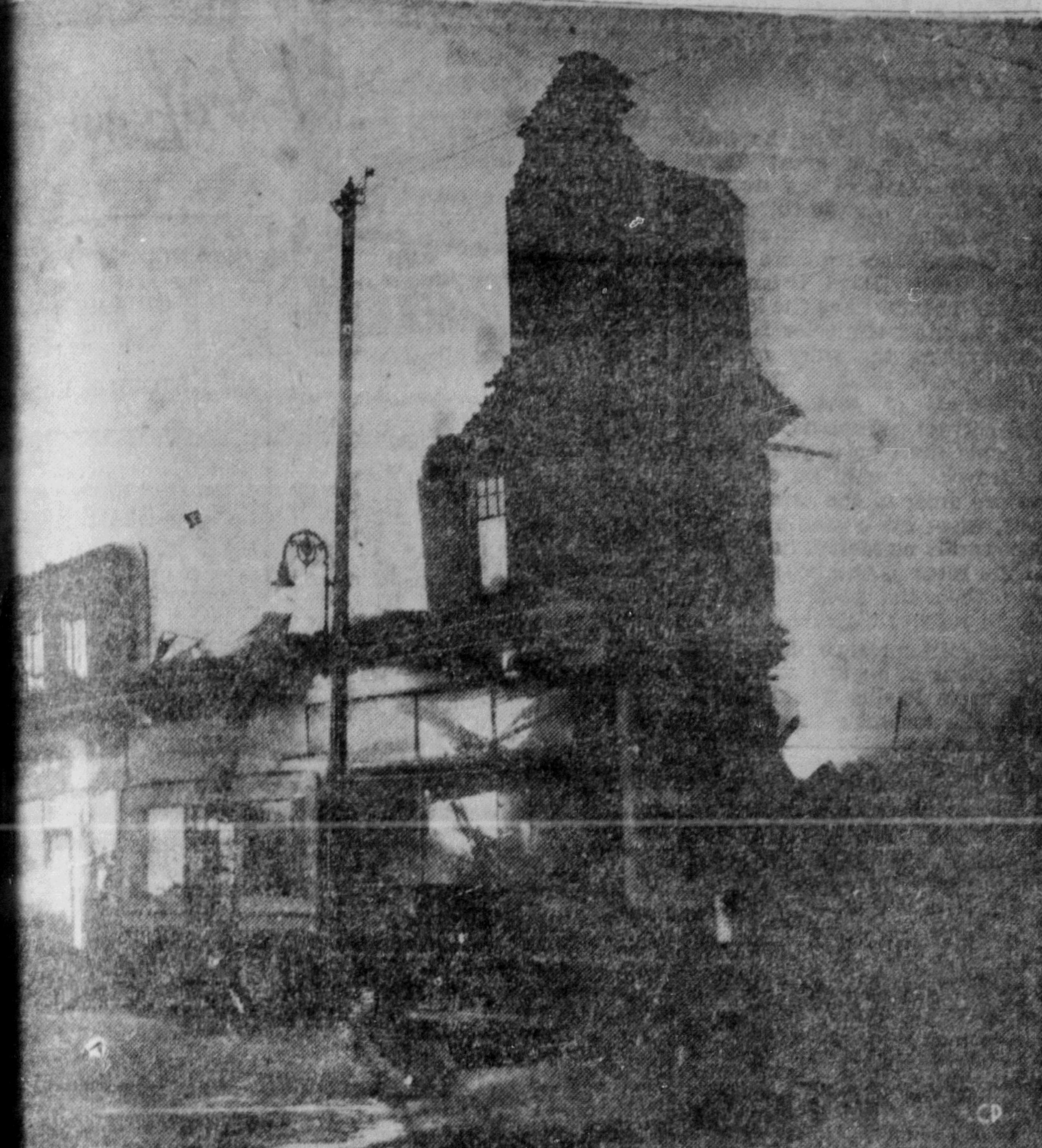
HOTEL BURNS—Two walls have fallen showing fire still raging through the ruins of the Hotel Burns at St. Thomas, Ont., which was destroyed by fire early Sunday morning. One man is believed to have perished in the fire. This graphic photo shows one corner of the hotel still standing. Damage was estimated at $300,000. (CP Photo)
