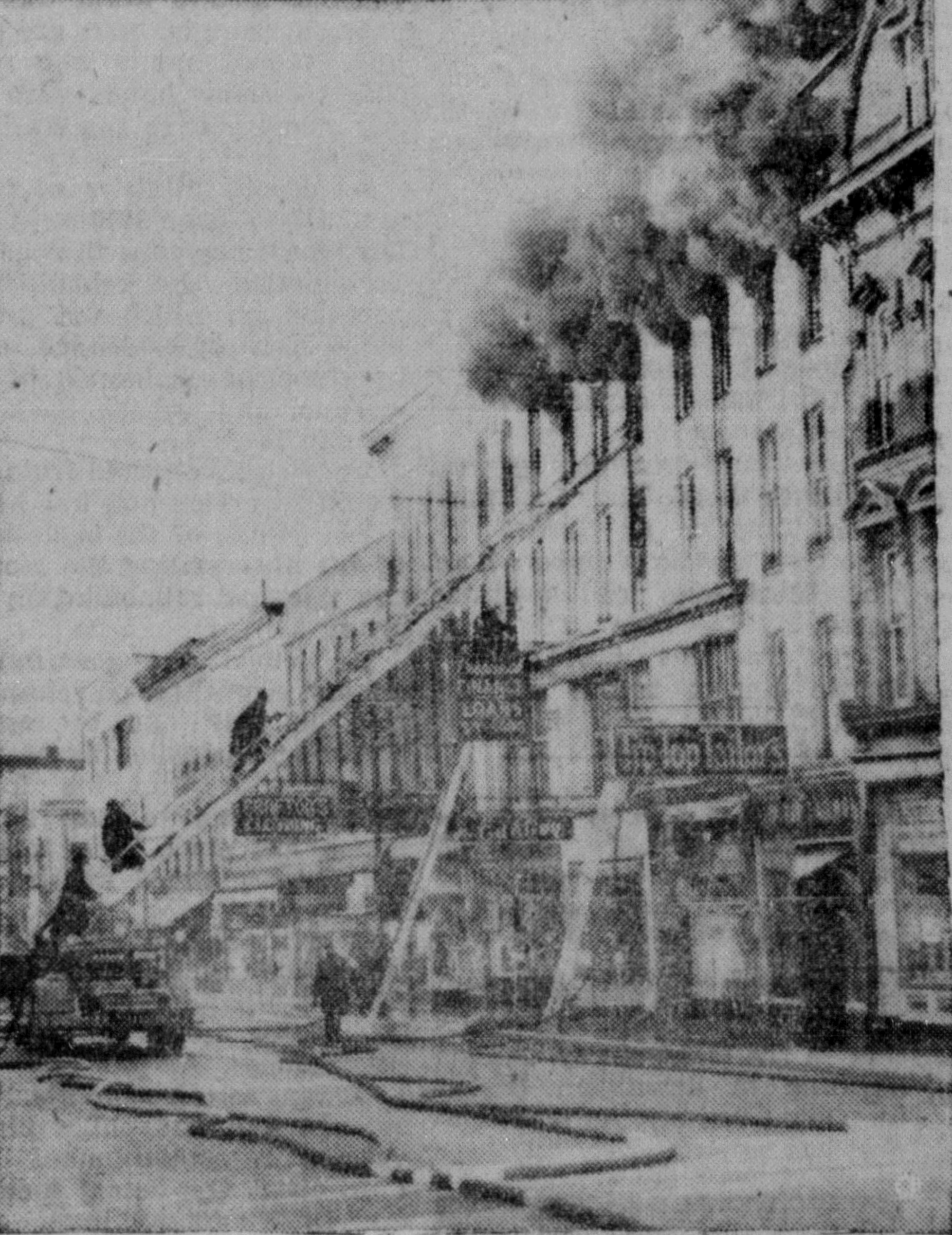
FOUR DIE IN FIRE —Three firemen and a volunteer were killed in this fire at Peterborough, Ont., when ceiling and floors collapsed. The building—in the centre of the city's business district—was a total loss. Damage was estimated at $300,000. (CP PHOTO)
