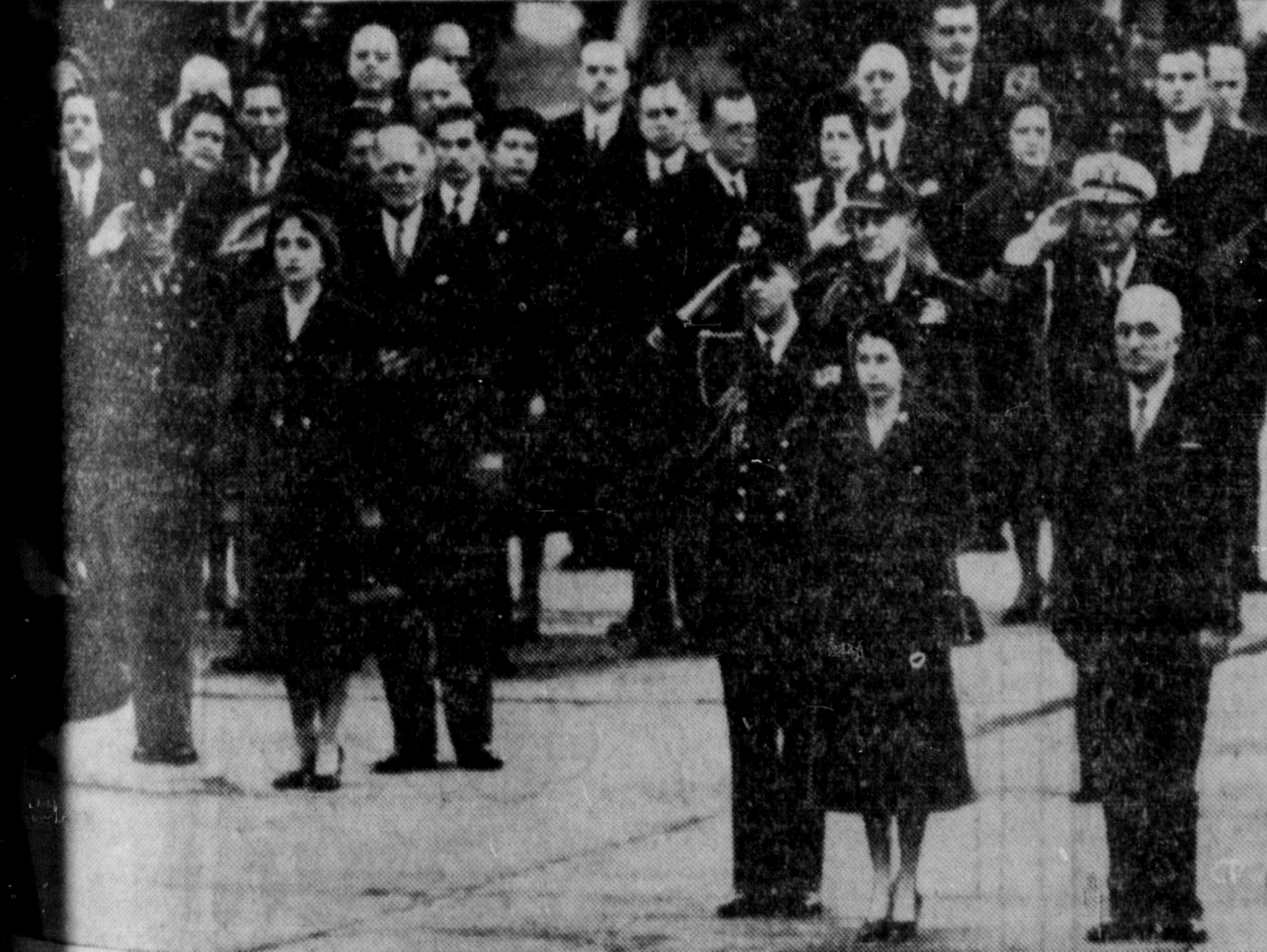
WASHINGTON AIRPORT—The official welcoming party stand at the salute during the arrival of the National Anthem shortly after Princess Elizabeth and the Duke of Edinburgh at Washington airport. The Princess stands between the Duke and President Truman. (Background). Mrs. Truman (far left) and daughter Margaret (third from left) stand with military and government officials. (CP from AP)
