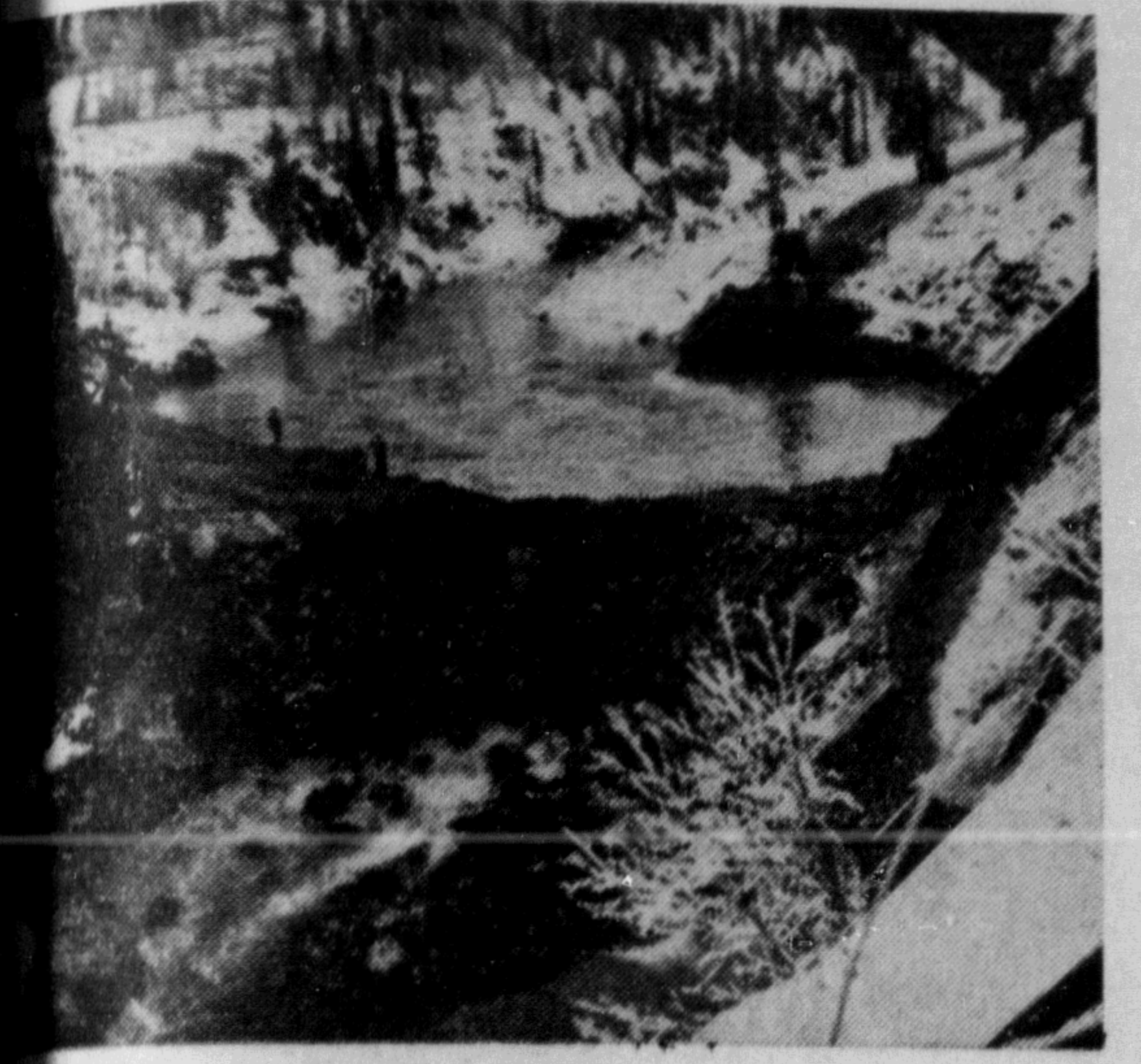
MAKO DIVERSION —Here is shown the cofferdam which was in connection with the diversion of the waters of the Nechako far in the interior south of Vanderhoof, into the western main river which will supply the Kitimat aluminum smelter.
