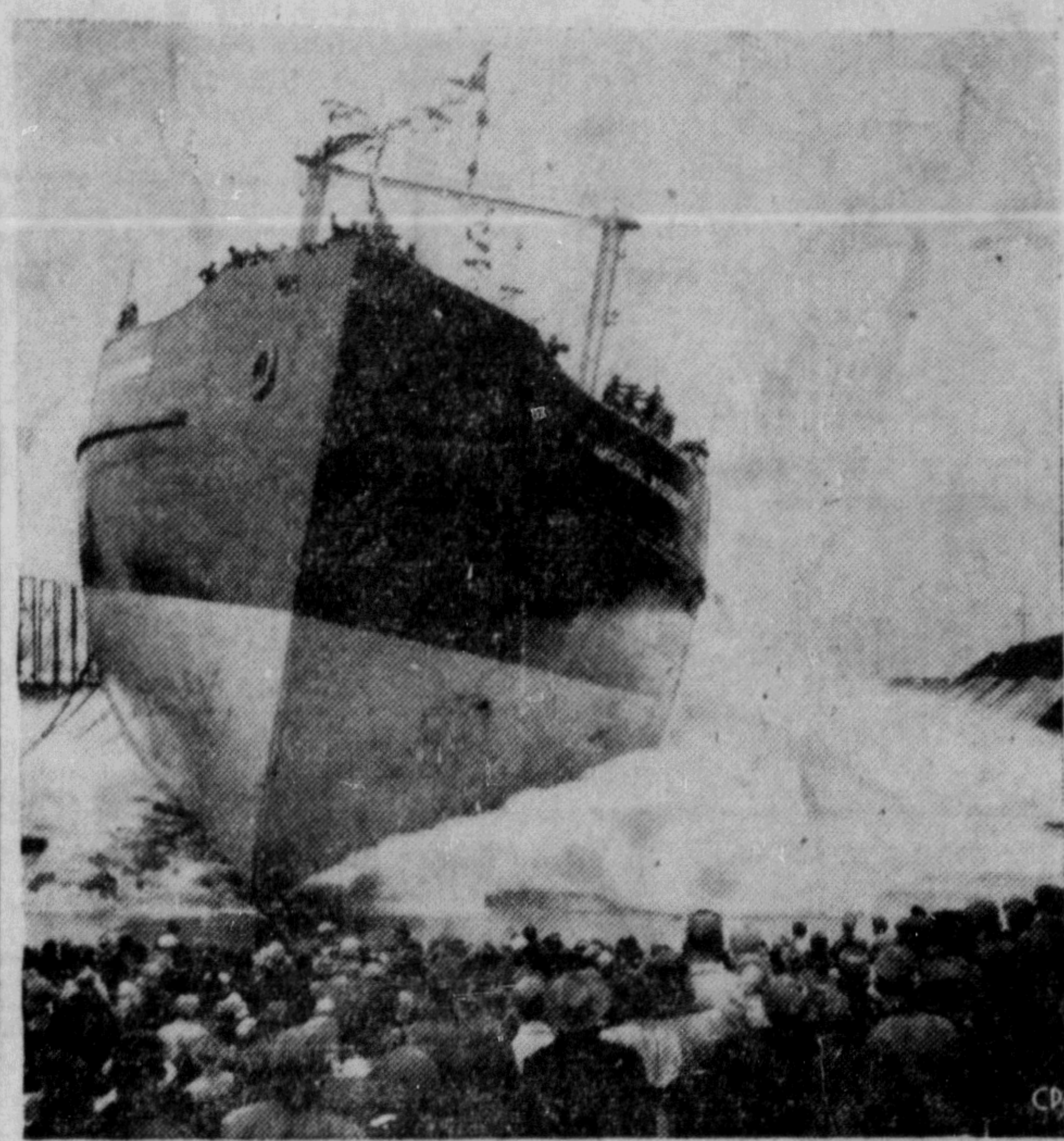
TANKER LAUNCHED—The Imperial Woodbend, 620-foot tanker which will carry Alberta oil to eastern refineries was launched—sideways—Wednesday at Collingwood, Ont. A huge backwash swept several spectators off their feet. Built for Imperial Oil Ltd., and named for an Alberta oilfield, she is a sister ship of the Imperial Leduc and Imperial Redwater, world's largest freshwater tankers. She will transport about 5,000,000 barrels a season. (CP PHOTO)
