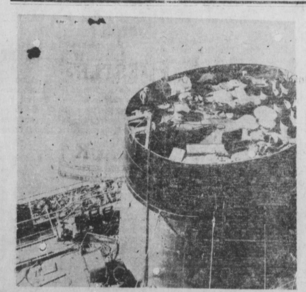
Top of funnel of new French motor-vessel Lafayette, showing sm oke tubes at rear, also ventilators sireen and smoke-stack staircas e. Also giving an idea of how complicated a smkoe-stack can be.
