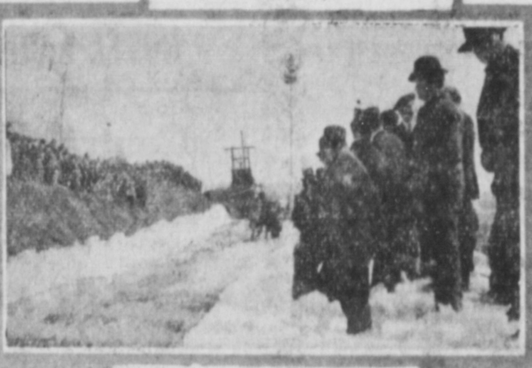
Track-layers making the last connection on the G.T.P. on Apr. 7, 1914, near Ft. Fraser
