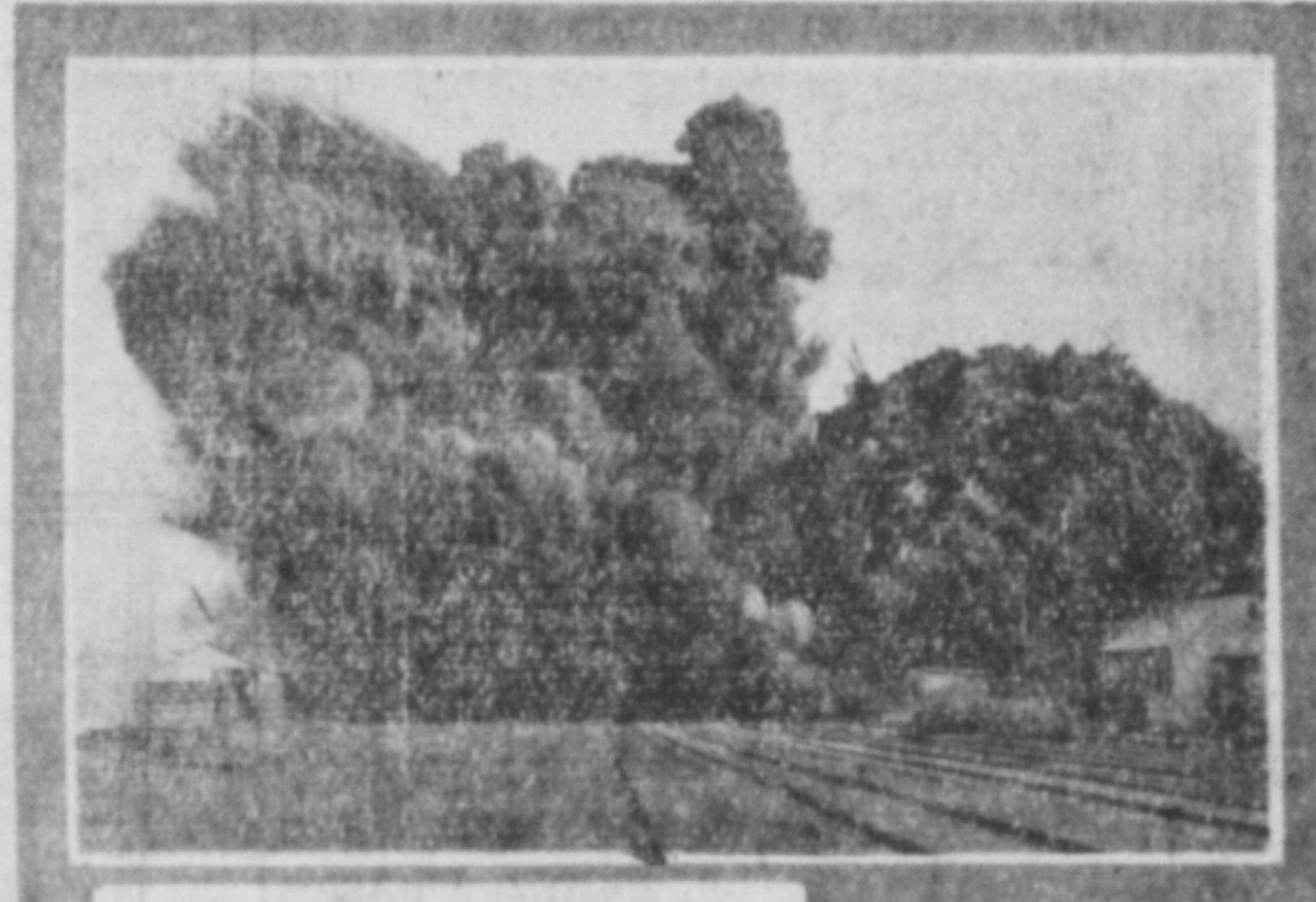
The last big blast on the Townsite Jan. 21, 1914
