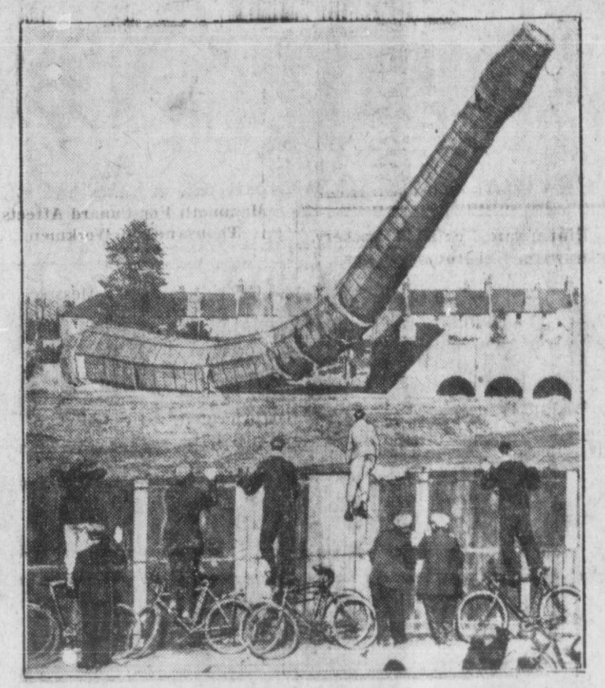
This 150-foot chimney at Tootin . England, is seen toppling with its 800 tons of brick just after a blast shook it from its base.
