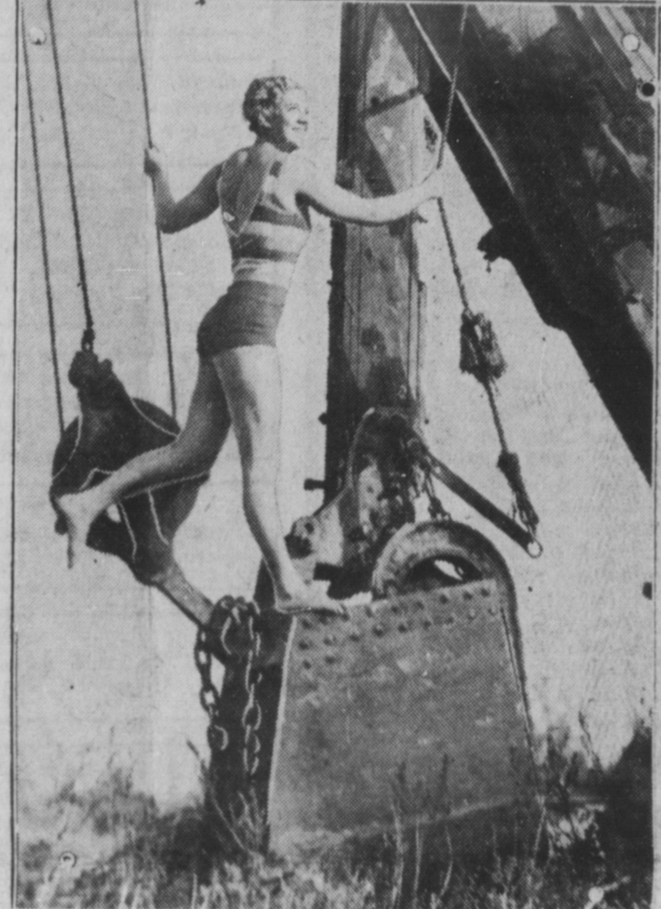
Georgia Coleman, world champion girl diver, pulls the switch of the steam shovel which is to excavate the ground for the new pool in Los Angeles where the Olympics will be held in 1932
