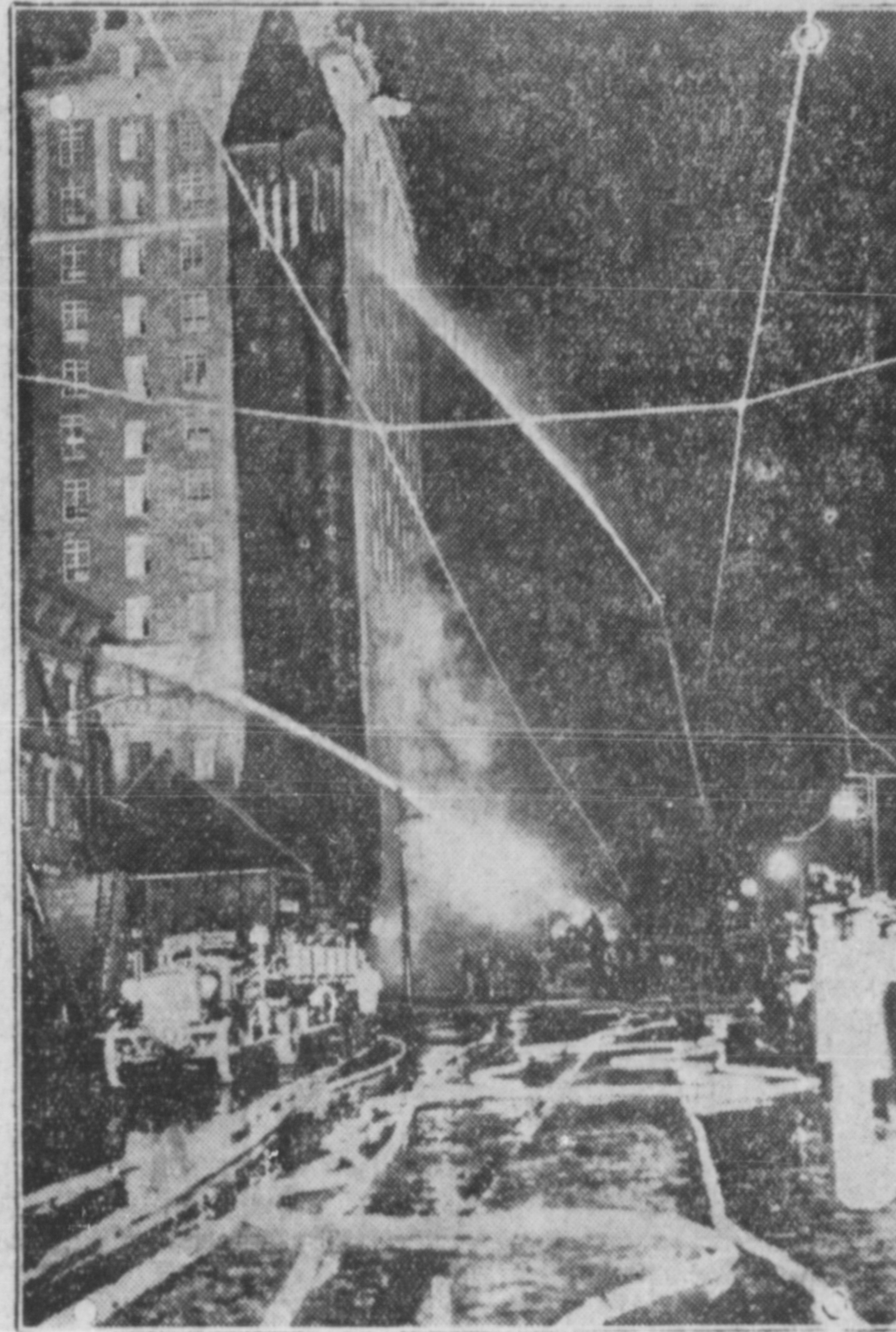
Firemen fighting devastating fire which wrecked Second Presbyterian church Newark N.J., causing damage estimated at $250,000. Four alarms called 22 fire companies into action.
