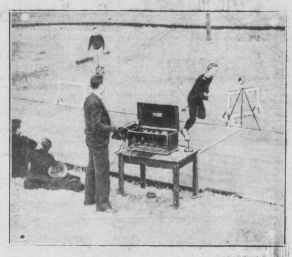
Haverford college students crossing finish line of new racing ray constructed by Edwin Speakman of Haverford, which projects beam of light across race track, registering running time to one one hundreth of second
