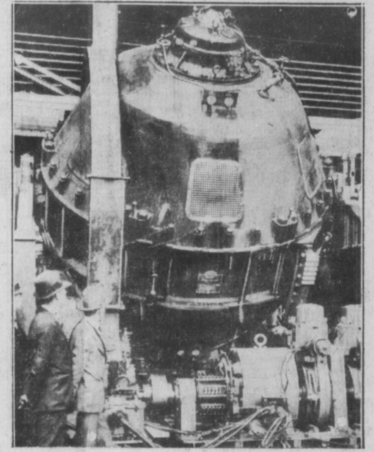
Boys play with tops—and so do men. Here is a giant 130-ton gyroscope stabilizer, anti-rolling device for ships, at South philadlephia works. Engineers say it will keep a vessel 450 long within two degrees of maximum roll.
