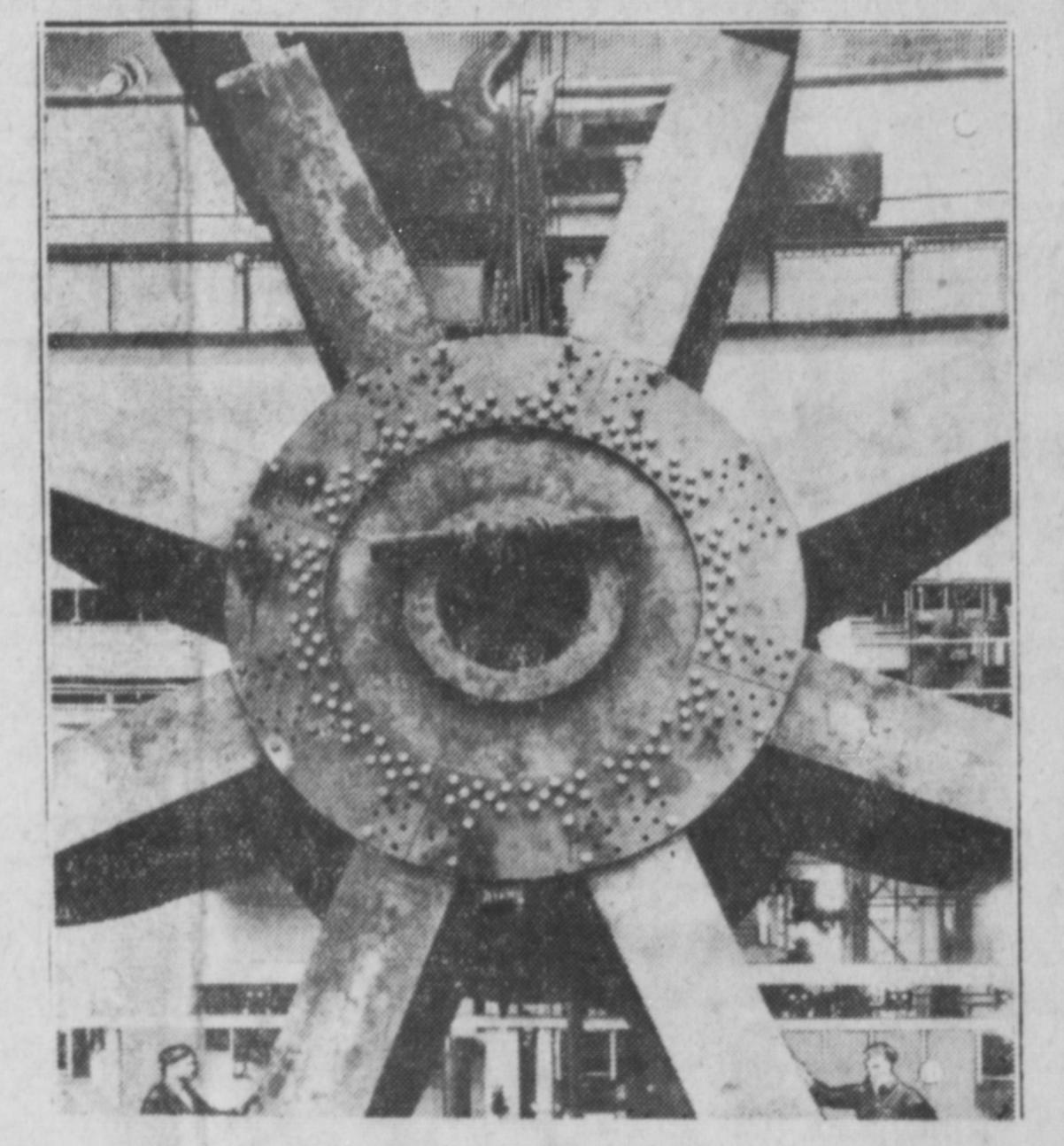
More power to the Soviets will be furnished by this giant waterwheel generator. The section weighs 92 tons and will be shipped from Schenectady to the Dneiper River station.
