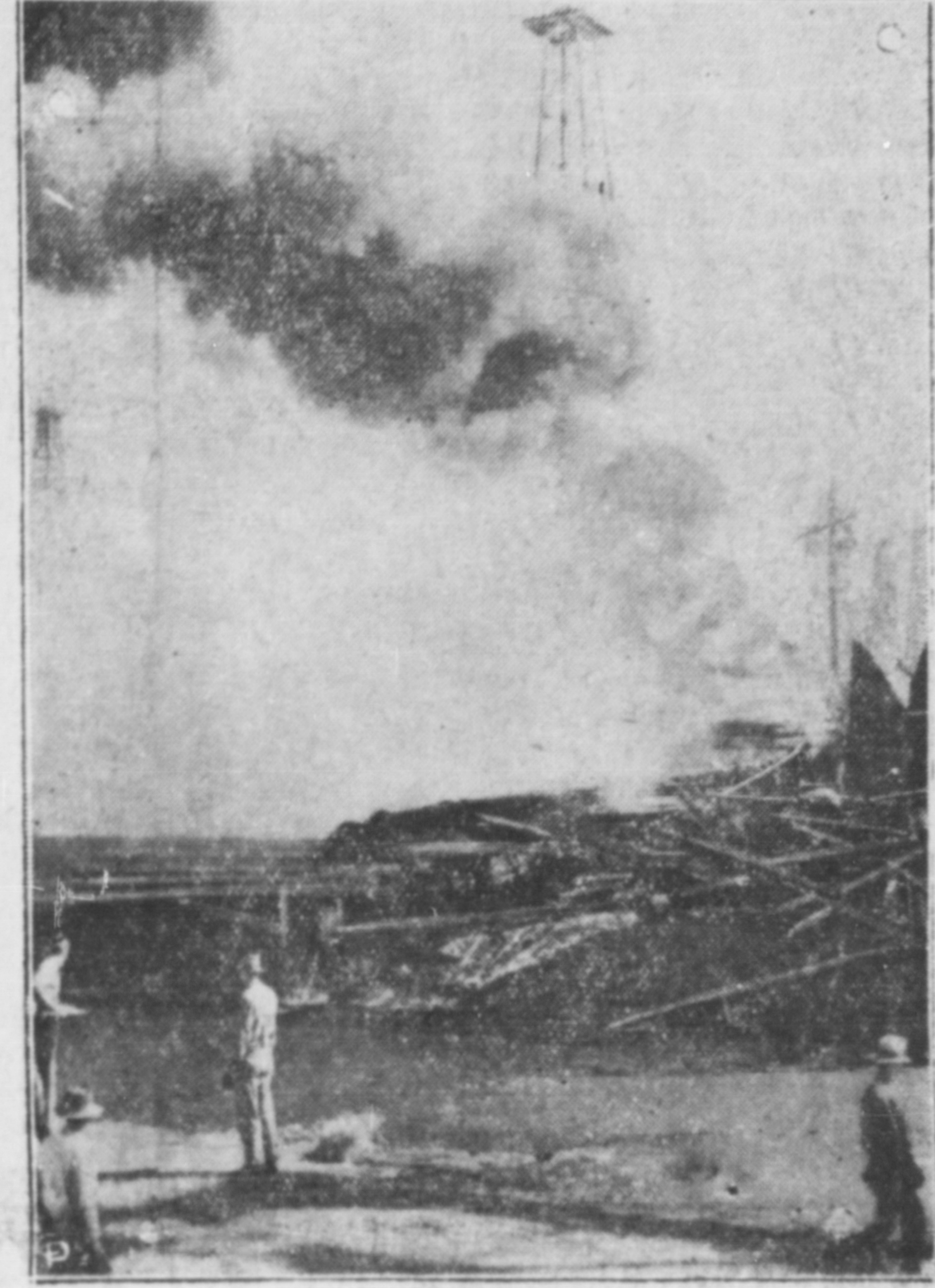
Photo shows oil fire at Huntington Beach, Calif., which originated at a rig near Fifteenth and Orange Streets, and was said to have involved two storage tanks and derrick and interrupted communication to the northern part of the field. All precautions were taken so as not to endanger the hundreds of oil well derricks in that vicinity. This was about the fourth major oil fire in the United States in a week.
