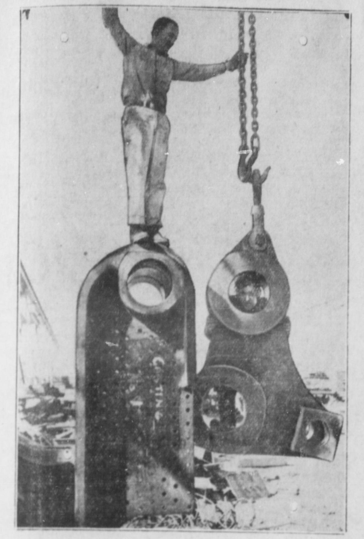
World's largest hinge by a dam site. That's not cussing, that's not cussing, that's straight fact. This hinge, cast of the finest steel, will support a weight of 2,200,000 pounds. On it will swing the huge gates of the Hoover dam.
