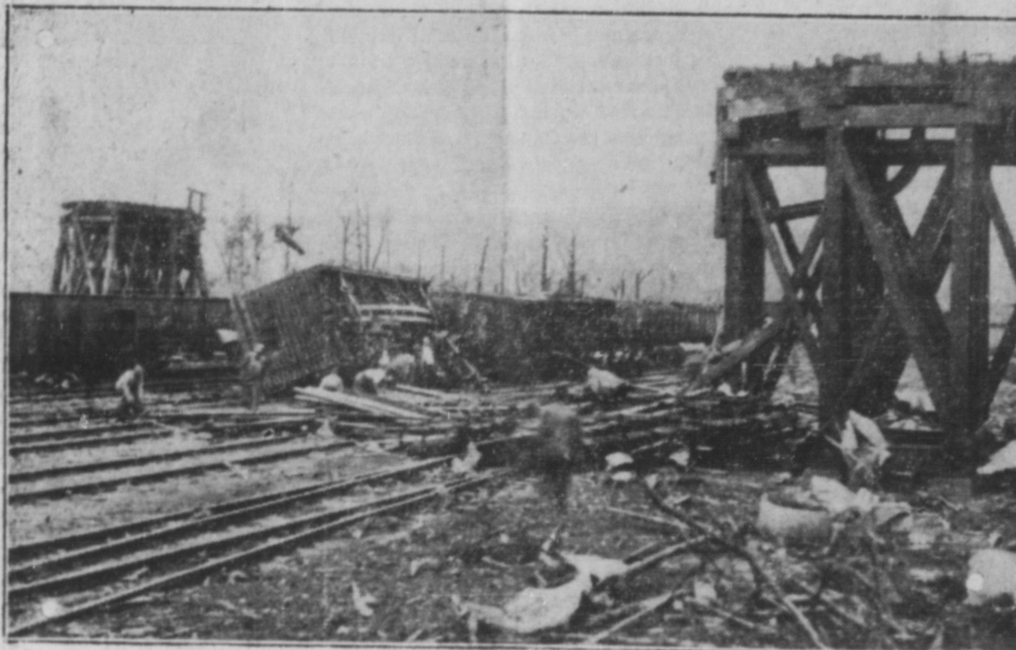
Freight cars on the Louisville and Nashville Railway at Helena, A. la., were tossed about and smashed by a tornado which swept through the mining town May 5, killing 13, injuring more than 100 and demolishing two-thirds of the town's buildings. At right is all that is left of a 50,000-gallon water tank
