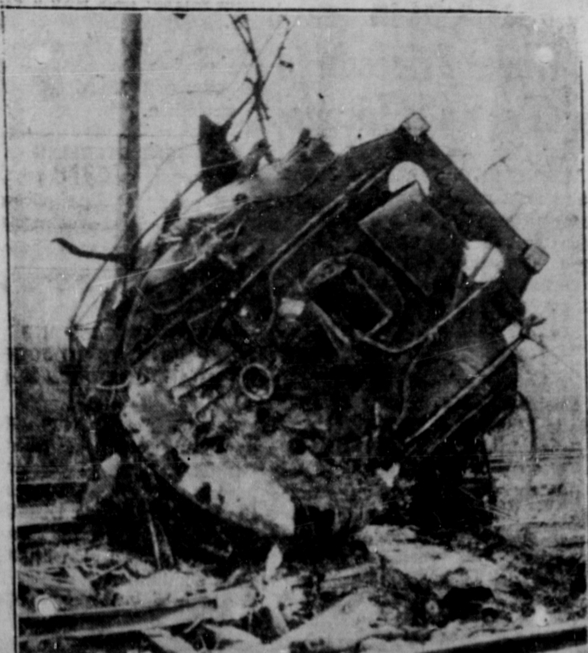
The wreck of an engine at Cedar Falls, Wash., that exploded when the boilers went dry, killing the engine watchman. A portion of the engine was hurled 150 feet.
