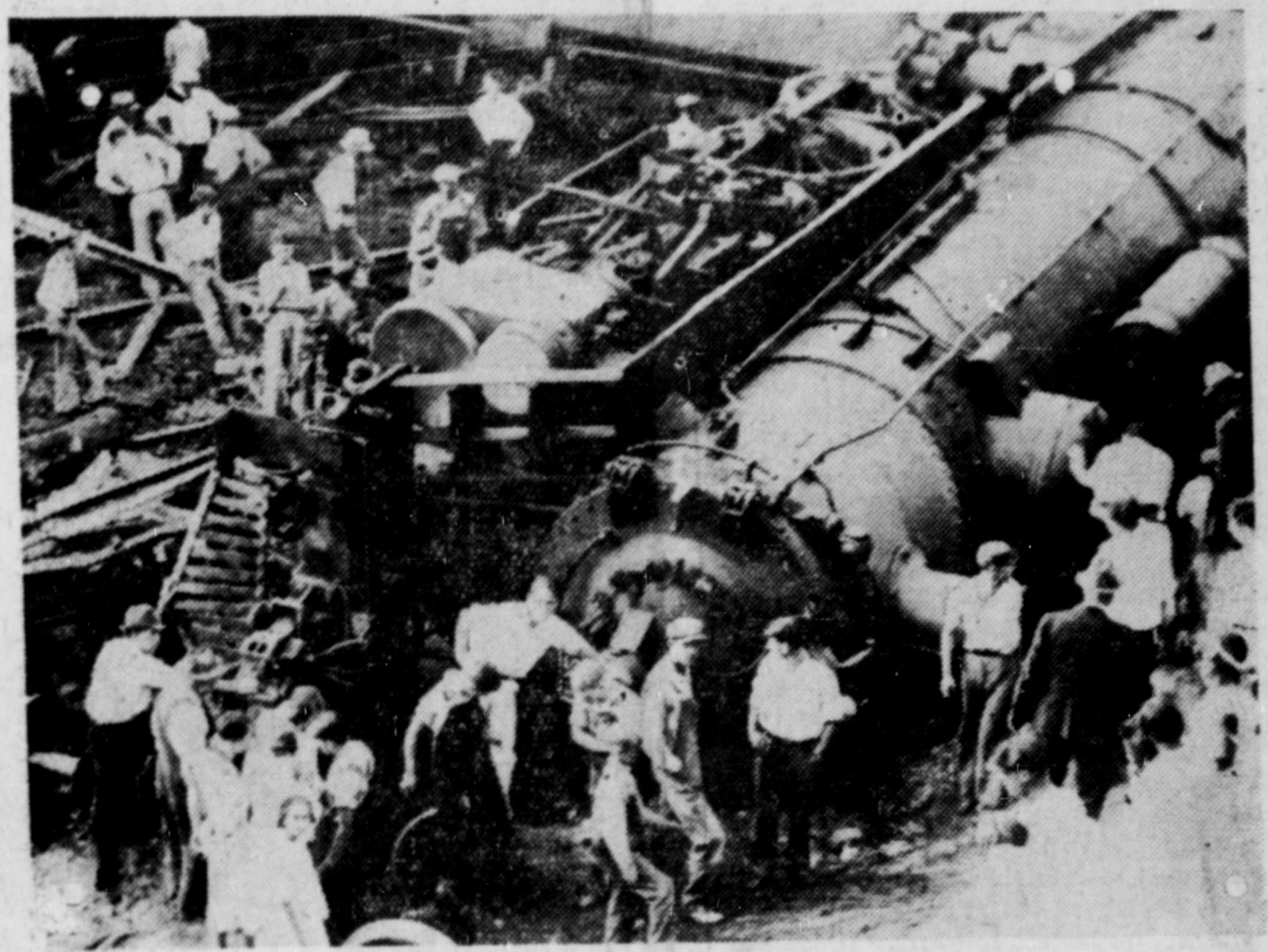
Authorities at Dora, Ala., believe this wreck of the engine of a fast passenger train, which was derailed near Dora while operating between Memphis and Birmingham, was caused by a small bolt placed on the rail by a small byy to have it "iron flat." Photo shows rescue workers at the scene. Engineer Tom P. Kelly was scalded to death, and Fireman Bert Davis was critically injured.
