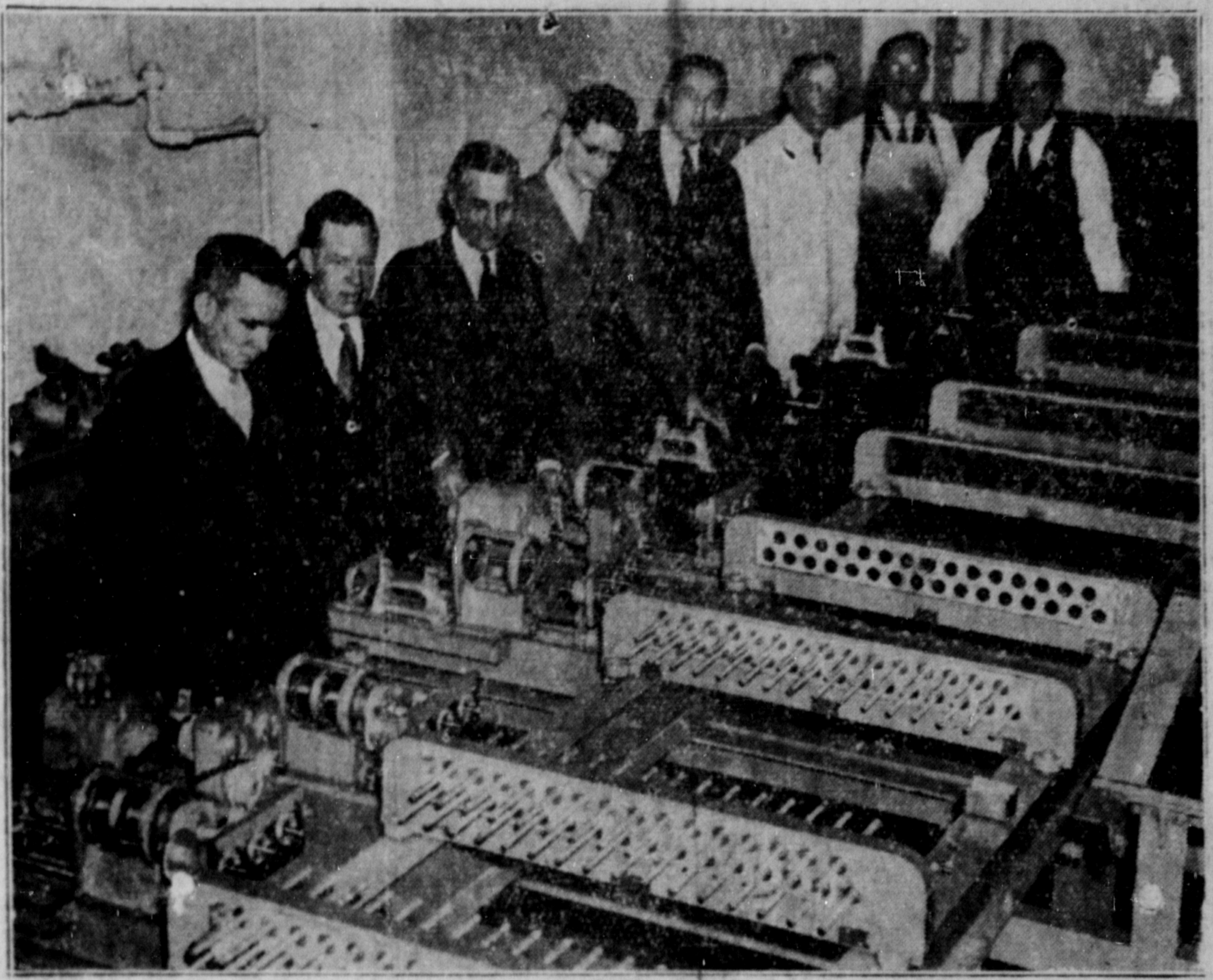
A group of civil works administration workers engaged in the construction of the differential analyzer, at the University of Pennsylvania, which will solve, in 15 minutes, mathematical problems that would take five experts four months to do.
